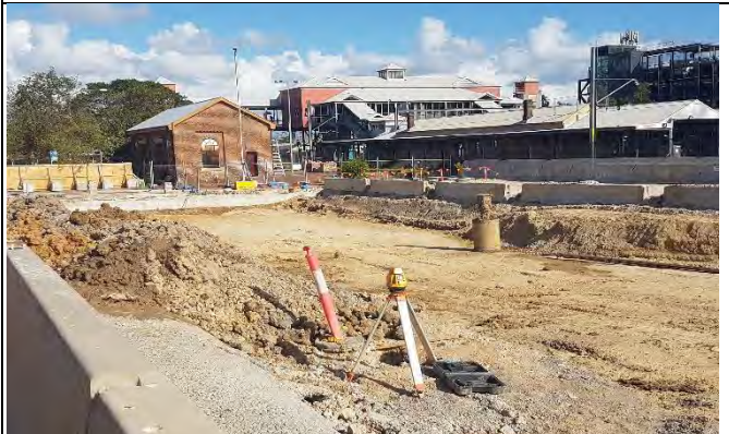
St Marys - View west from Station pf completed western piling pad.
