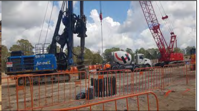
Orchard hills– view northwest of piling works in dive area south of Lansdowne Rd .
