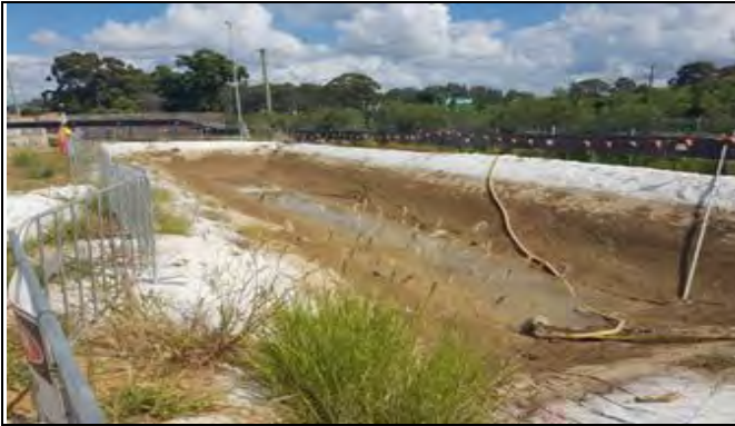
Claremont Meadows – View southwest along Great Western Highway of basin in operation and emptied
