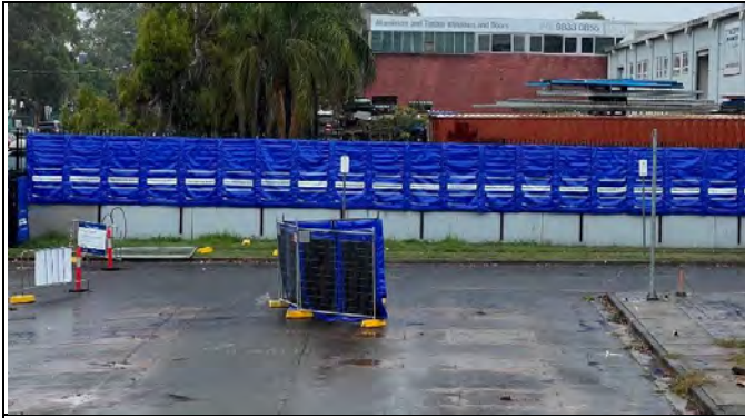
Eastern site boundary – Acoustic blankets installed and a movable noise hoarding for specific tasks or items of plant
