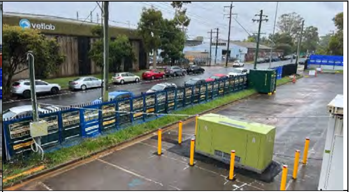
Northern Boundary - Noise blankets have been installed along the fence on Harris Street
