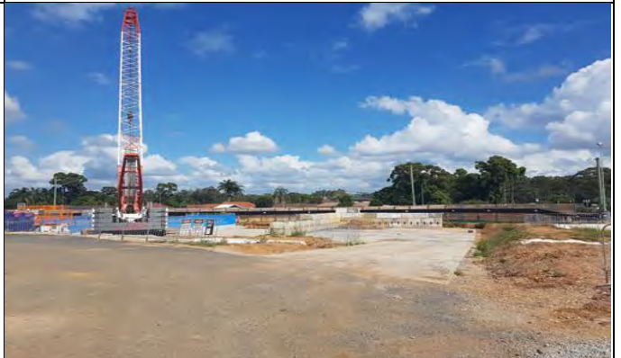
Claremont Meadows view southwest – Shaft excavation spoil storage area
