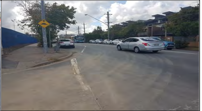
St Marys looking southeast from Gidley St: Negligible tracking noted at exit to Philip St
