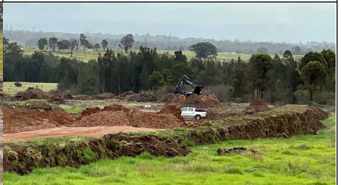
M12 to Cosgroves Creek - Recently cleared vegetation is being mulched or retained for future reuse
