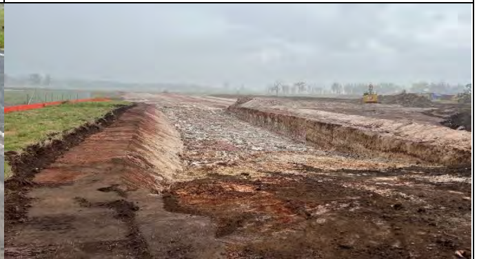
Luddenham Station – earthworks have commenced
