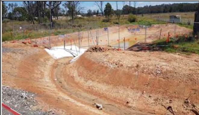
Bringelly Services Facility view north west–. Sed. Basin in operation and emptied
