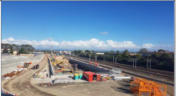
St Marys looking west - General view, with eastern station box in the foreground and piling at western extent.
