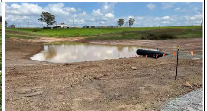
Elizabeth Drive - Pipes installed across the haul roads to allow flow from the M12 site to existing farm dams
