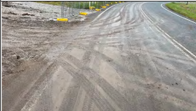
Luddenham Station - Mud was tracked out of the site access track.
