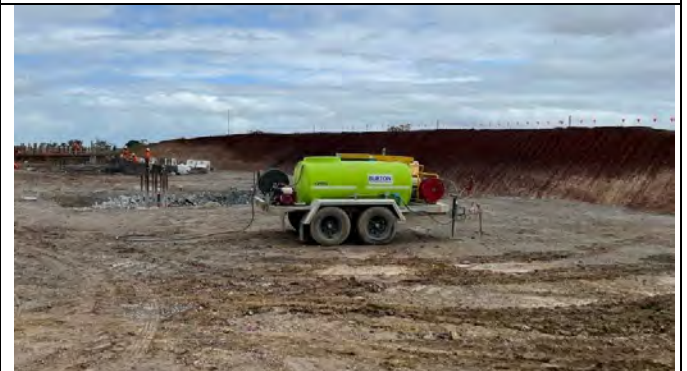
Elizabeth Drive - Water tank used to collect and reuse water within the site
