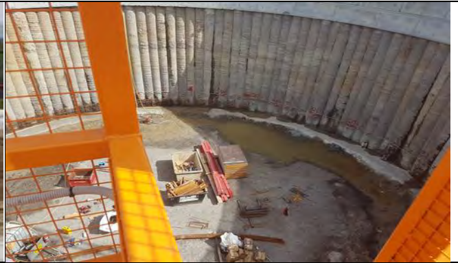
Claremont Meadows– Shaft excavation ring beam FRP
