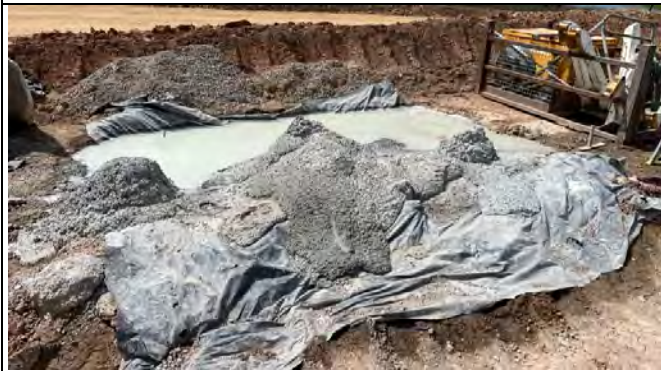
Elizabeth Drive – the concrete washout was inadequate and needed rectification.
