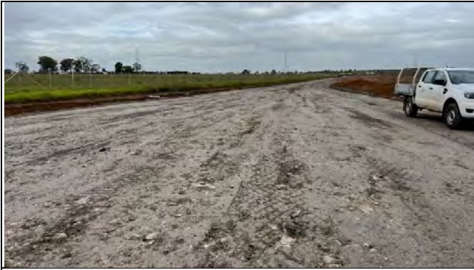
SMF - Sandstone has been placed along the access tracks to create all weather tracks
