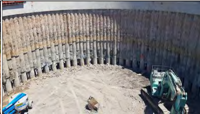
Bringelly Services Facility – Services shaft bulk excavation.
