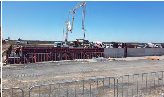
Aerotropolis : Station box north capping beam and upstand FRP.
