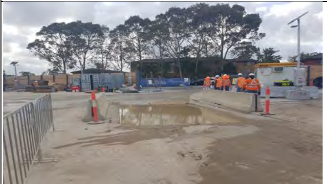
St Marys Main (Station Plaza) Laydown area : Eastern rumble grid / wheel wash in operation and effective.
