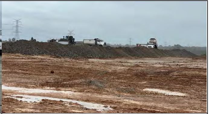
SMF - Sandstone material transferred from the site at Patons Lane to the SMF during construction hours
