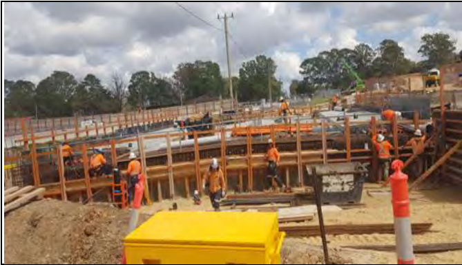
Orchard Hills view west – Bridge deck and abutting walls FRP ongoing at Lansdowne Rd bridge over station box.
