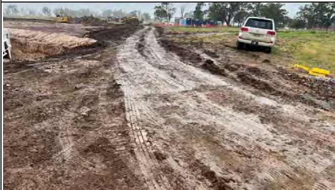
Luddenham Station – Earth access track needs to be stabilised all weather access track
