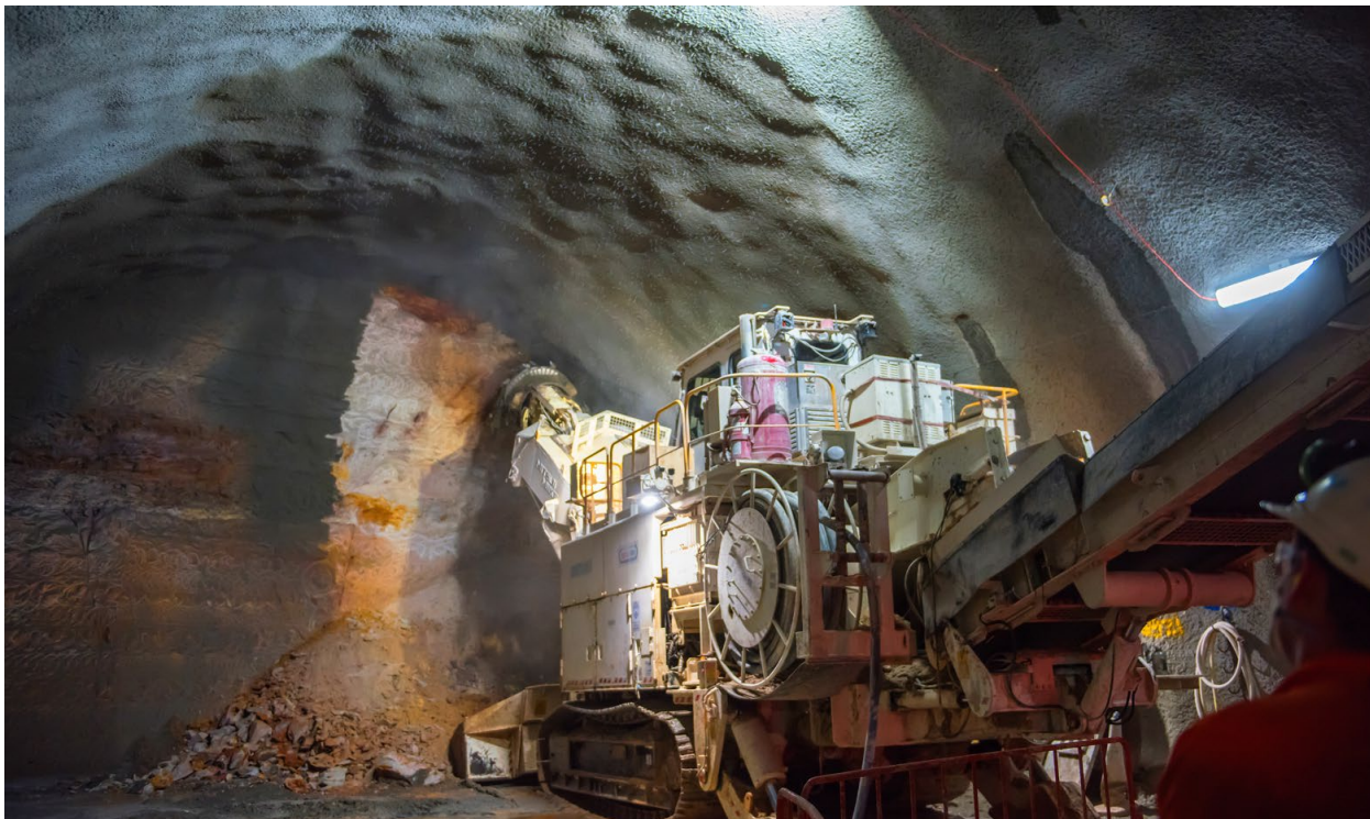
Figure 1 Roadheader used in tunnelling
