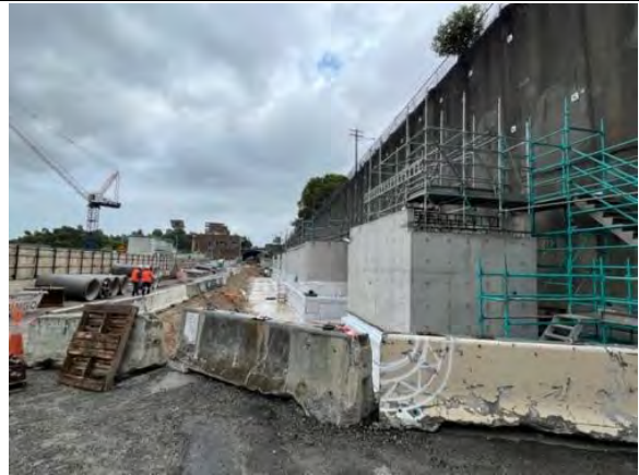
Ongoing installation of the ventilation pods in Zone 4
