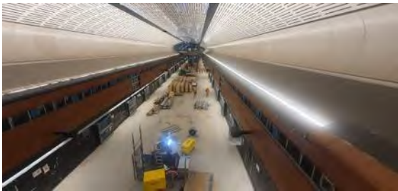
Station Cavern: Façade installation above trackway, station fit out and GRC panels progressing
