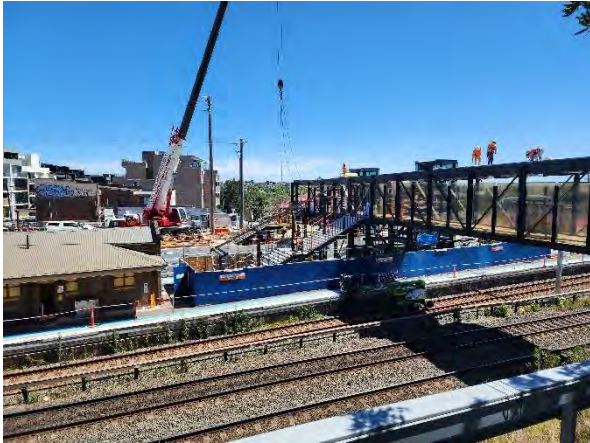
Dulwich Hill: Footbridge stairs and roof installation
