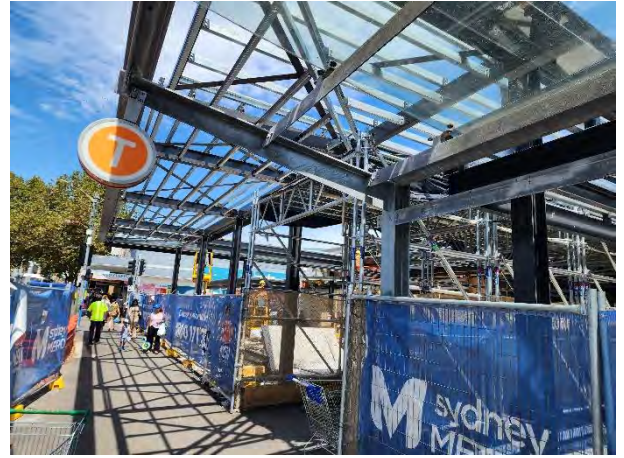
Campsie: Concourse structural steel installation
