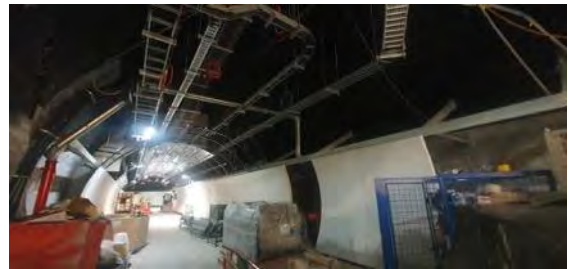
Public Adit: GRC panel installation progressing
