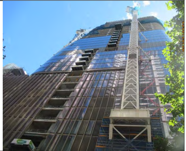
Martin Place North: View from street level on Elizabeth Street. SSI works top out at Level 7. Use of work zone on Elizabeth Street to deliver materials using the tower crane attached to the building
