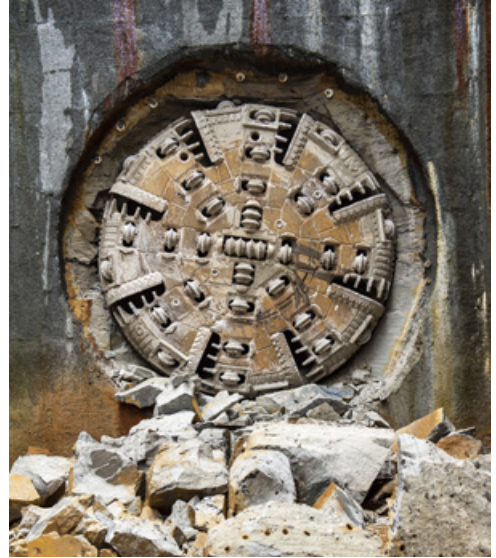
Tunnel Boring Machine (TBM) Mum Shirl Barangaroo breakthrough.
