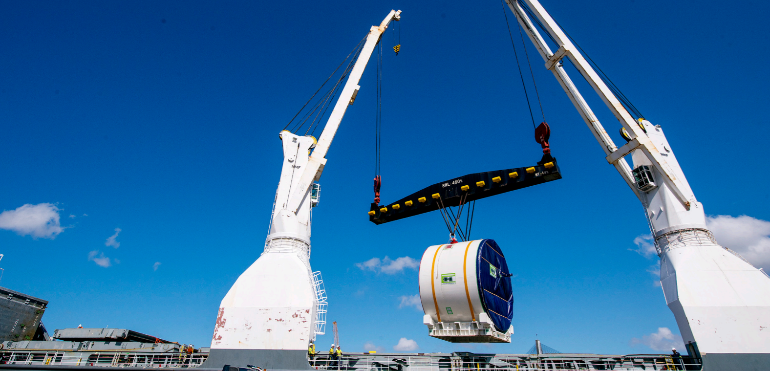
Tunnel boring machine arrival at The Bays Station site.
