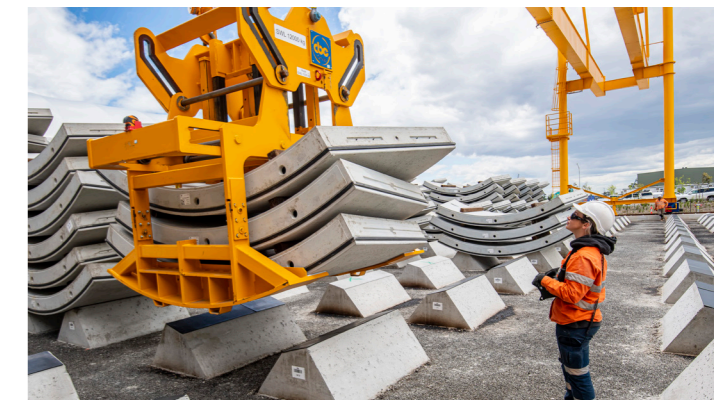
Concrete segments at the precast facility at Eastern Creek.
