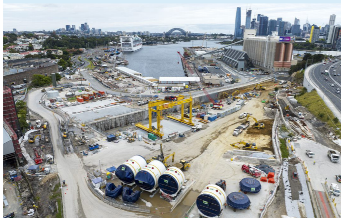
Construction progress at The Bays Station site.
