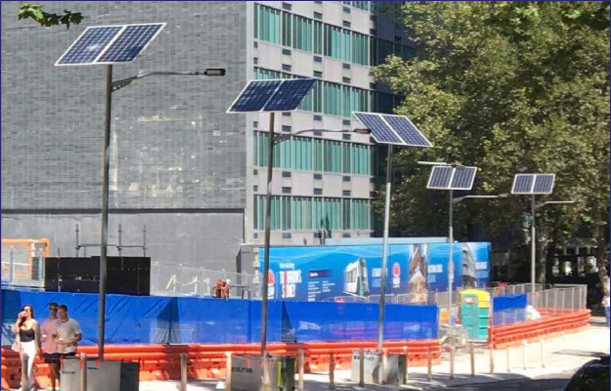
After removal of street lights, five temporary relocatable solar-powered lights were installed adjacent to the Victoria Cross site. These lights have saved more than 1000 kilograms of carbon dioxide emissions (kgCO2-e) to date.
