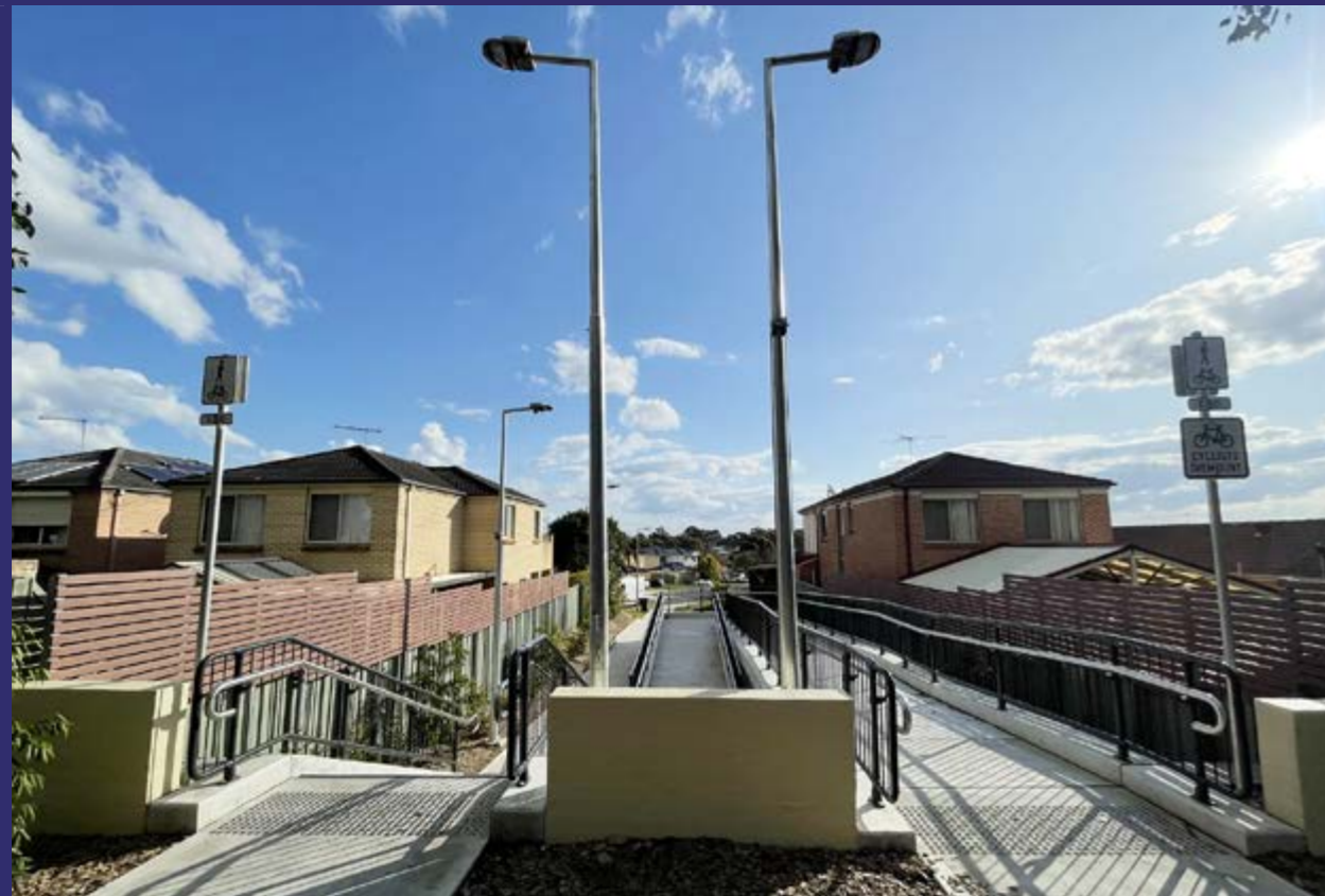
The new Glenwood Pedestrian Link.
