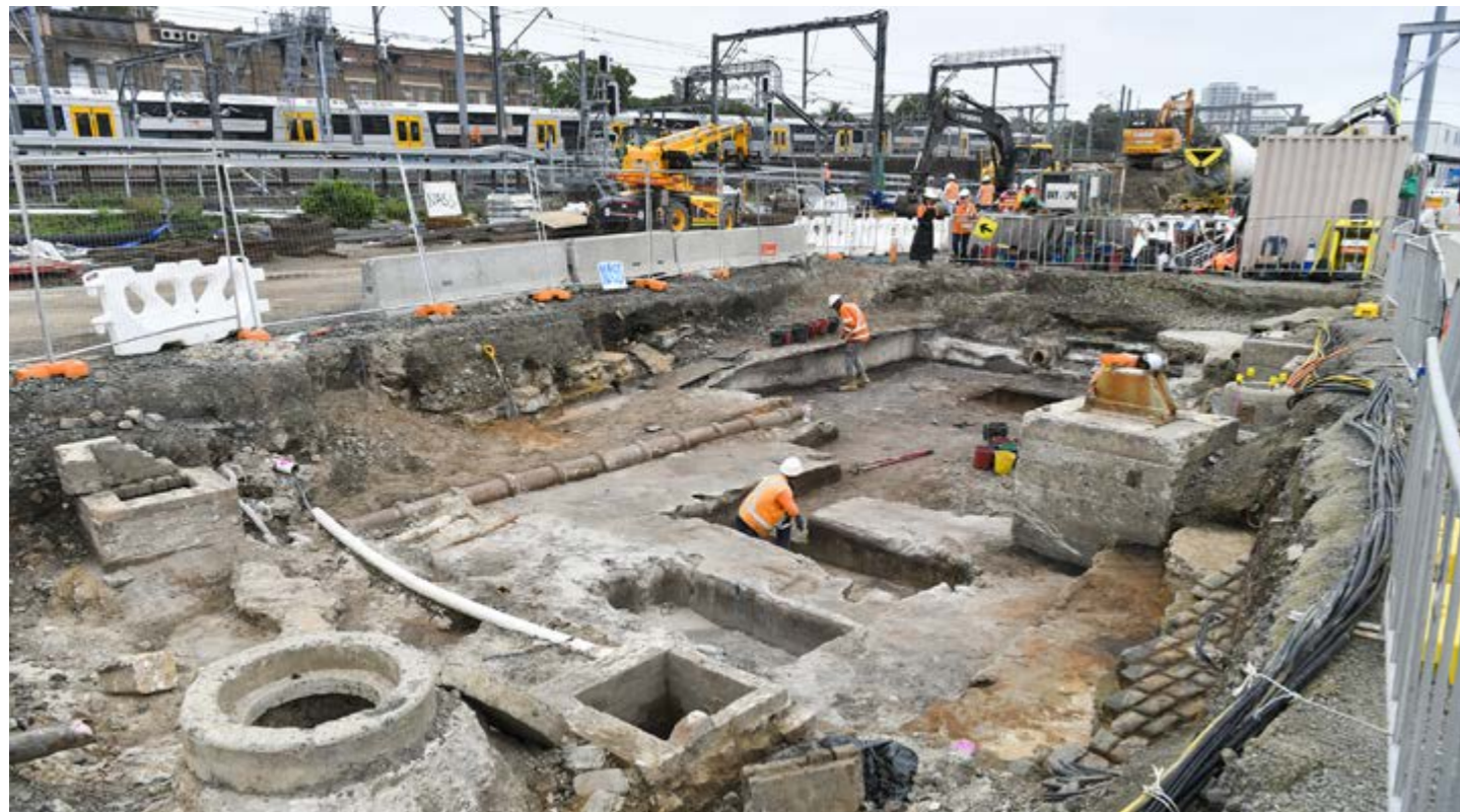
Excavation at Central Station.
