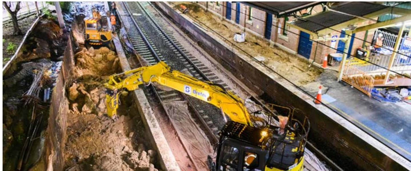
Work to upgrade and convert the tracks and platforms to Sydney Metro standards on the Bankstown Line (Canterbury Station).
