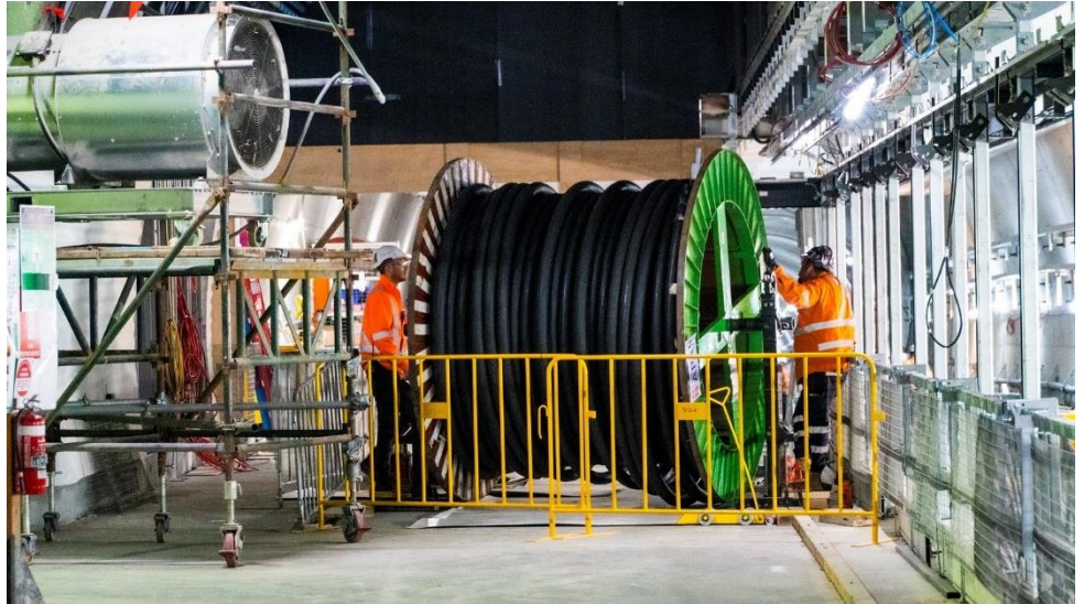
Workers at Pitt Street Station are installing 80 kilometres of cables, including high voltage cables to power the station and trains.
