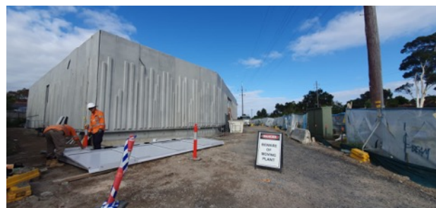
Dulwich Hill TSS - Preparatory works on steel roofs for transformers underway.
