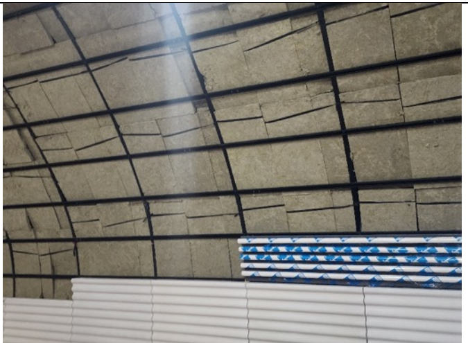
Adits: Ceiling Insulation and cladding installation.
