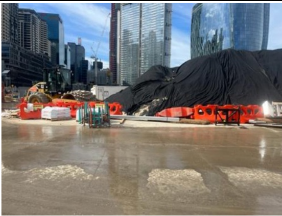
Stockpile and dust suppression via water cart ongoing; maintenance of controls required
