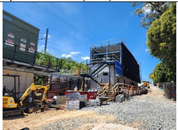
Hurlstone Park: MSB cladding installation
