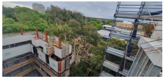
VCN: View of Slip form from Level 4 of VCN. Slip form (currently) at Level 3.
