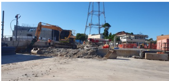
CDS (previous Acoustic Gantry Shed area): Concrete surface removal works underway,
