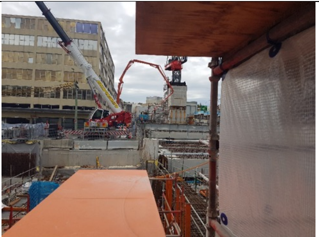
Clarke Lane South - Clarke Lane South, used under ROL for concrete pump, with new Tower crane 3 on the right
