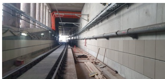
Northern Dive: Installation of dampeners (acoustic panels) on section of Northern Dive wall and track progressing.
