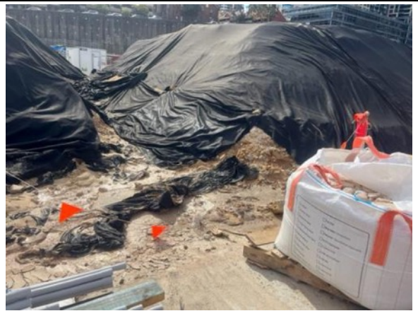
Stockpile and dust suppression via water cart ongoing; maintenance of controls required
