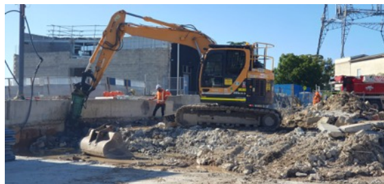
CDS (previous Acoustic Gantry Shed area): Observed dust suppression (operator wetting down the works area) during concrete surface removal works.
