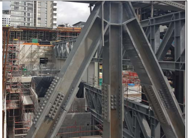
Site A B1 to L1 elevation looking north: Concourse area pre-assembled steel trusses in place
