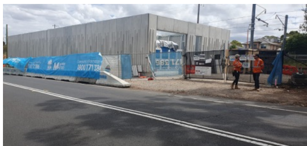
Punchbowl TSS: Remainder of façade installation scope completed under OOH#269.
