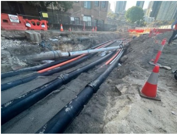
Completion and backfill of condensed water system in Zone 5 (Nawi Cove)
