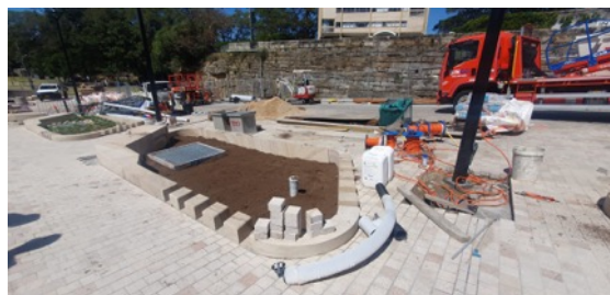
Blues Point Road – Streetscaping worksite: Finalising raingarden installation.
