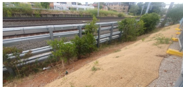
Campsie TSS: Batter trimming and stabilisation works progressing along the batter (track side).
