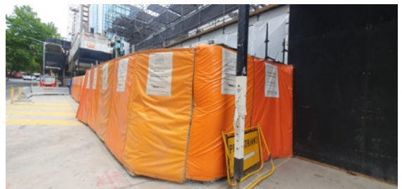
VCS – Miller St: Noise blankets installed appropriately around stormwater worksite on Miller St. No works at the time of inspection.
