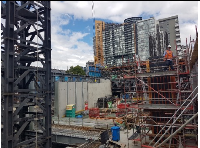
Site A view north: Level 1 FRP and Level 0 pre-cast interior walls
