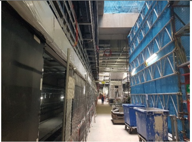
Platform (B5): Platform sliding doors and screen installation
