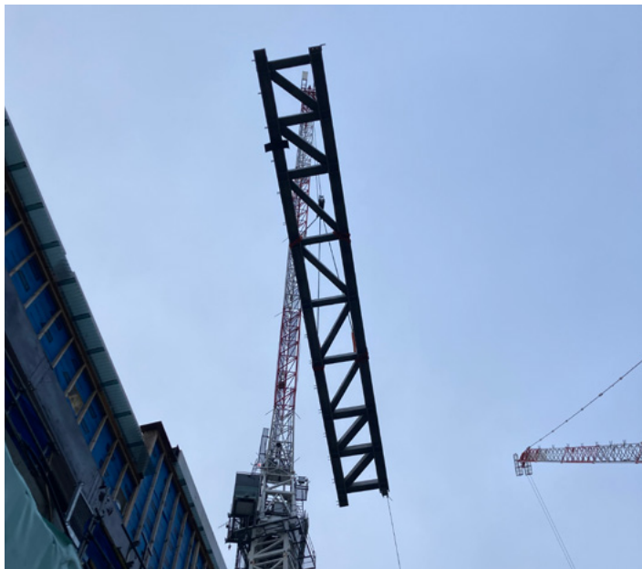
Installation of the transfer beam into the south site.
