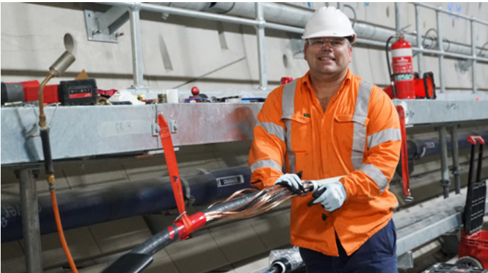
Workers laid two 11,000 volt power cables in the tunnels between Artarmon and North Sydney as part of the permanent power supply for Victoria Cross Station.
