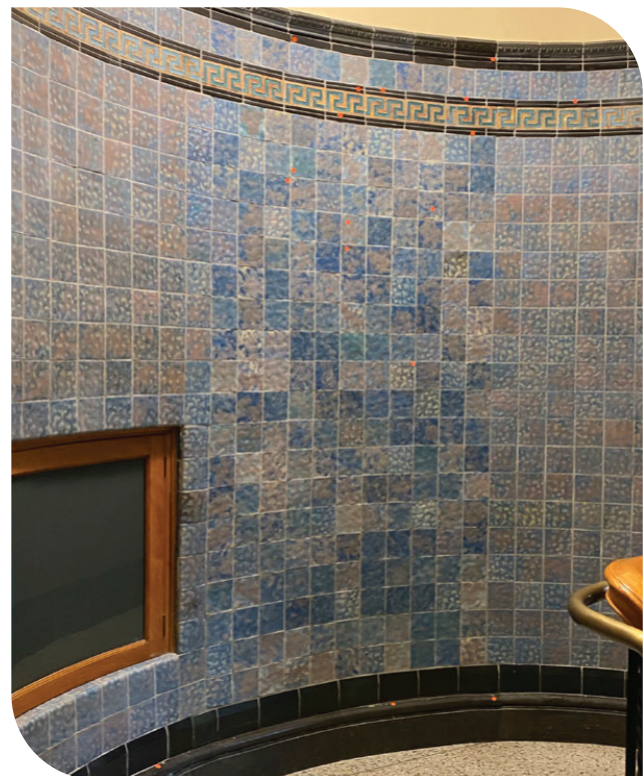
Infilled wall with salvaged and new.
