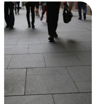
Austral Black granite pavers are specified for general footpaths and station entrances
