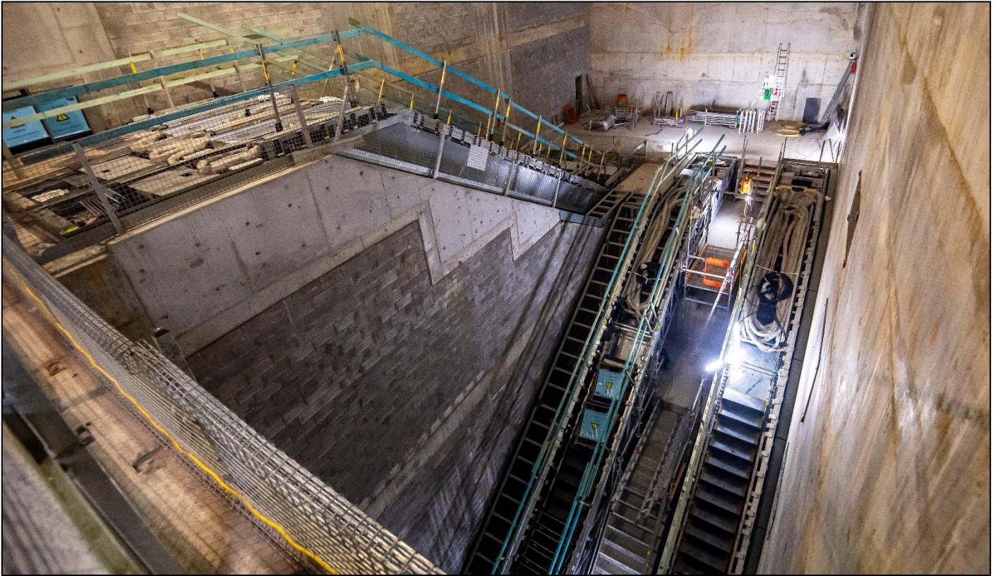
Escalators have been installed at the Pitt Street station south site.
