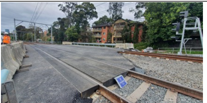
Northern Connection - Drake Street (rail corridor) - Hi-rail pad installed during the October Shutdown period.
