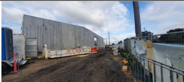
Dulwich Hill TSS - Façade panels largely installed in the October shutdown period with minor section remaining.
