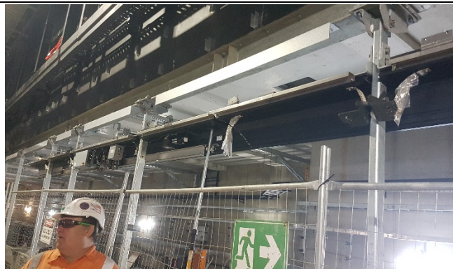
Level B5 - Platform Sliding Door mechanisms installation.
