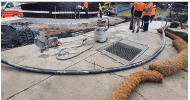
Blues Point Road – Streetscaping worksite: Saw cutting of existing concrete pavement; with vacuum observed for slurry management.
