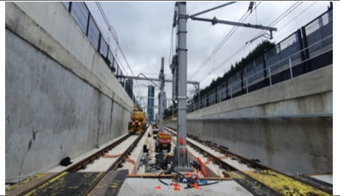
Northern Connection - OHW installation in Northern Dive section.
