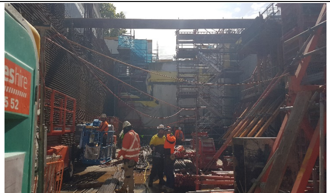
Site C view east– Perimeter wall shuttering and FRP
