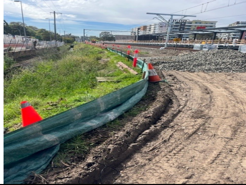
Bankstown Station: The sediment fence between the works and the North Terrace culvert had not been installed properly, increasing the risk of sediment entering the culvert during the next rain event. Controls were fixed prior to the next rain event.
