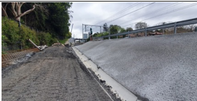
Northern Connection - Brand St (rail corridor) - cess drainage and batter shotcreting works undertaken during October Shutdown period.
