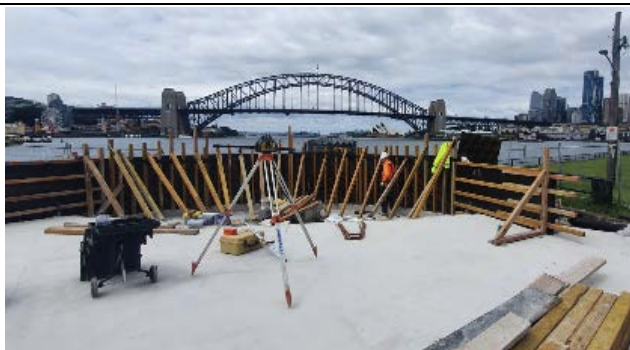
Blues Point Road – Streetscaping worksite: Formwork for Horseshoe Wall (Wall 1) in progress.
