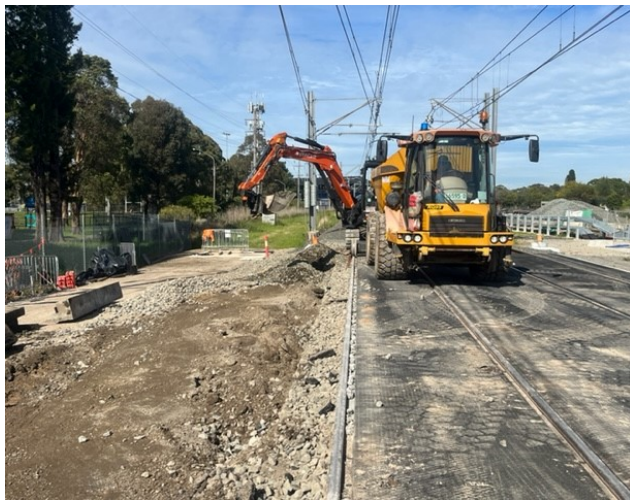
Loftus Street, Campsie: Ballast reconditioning was underway adjacent to the hi-rail access pad
