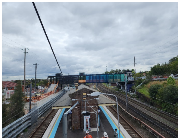
Dulwich Hill: Installation of the pedestrian bridge, stairs and lift shaft.
