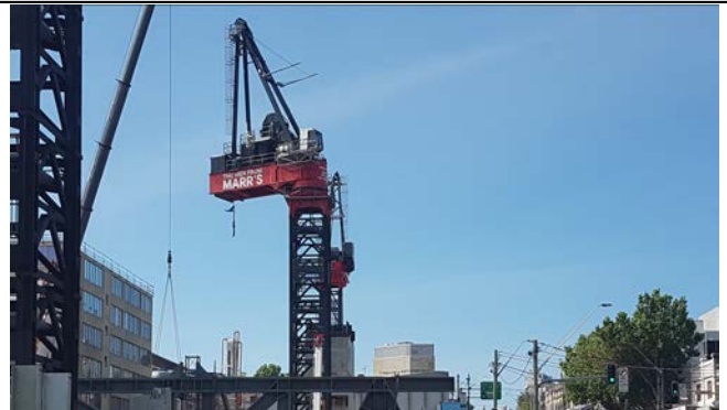
Site B (South) – TC 1 disassembly with replacement TC 3 assembly on Jump form at Level 2 beyond (background).
