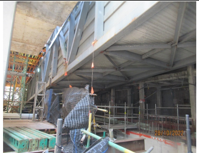
Martin Place Pedestrian Bridge: To be removed once pedestrians moved to new crossing within the MPS site
