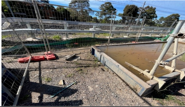
Belmore Triangle: One of the two slurry bins was full with risk of uncontrolled release with predicted rain. Water was pumped to another bin with additional capacity.
