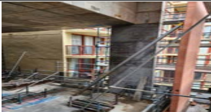
PSS - Level 5 pre cast façade panel installation adjacent Princeton Apartments.
