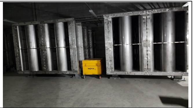
Over-track Exhaust: extraction fan plenum.
