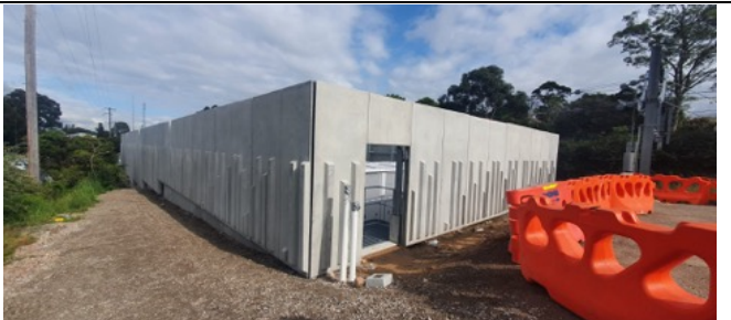
Canterbury TSS - Façade panel installation completed in the October shutdown period.
