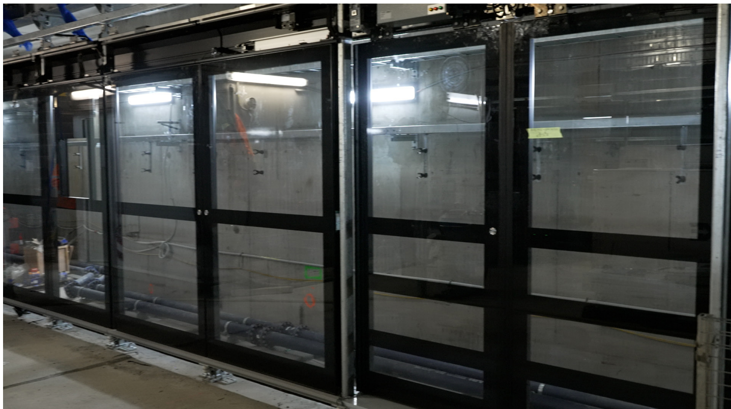
Installation of platform screen doors
