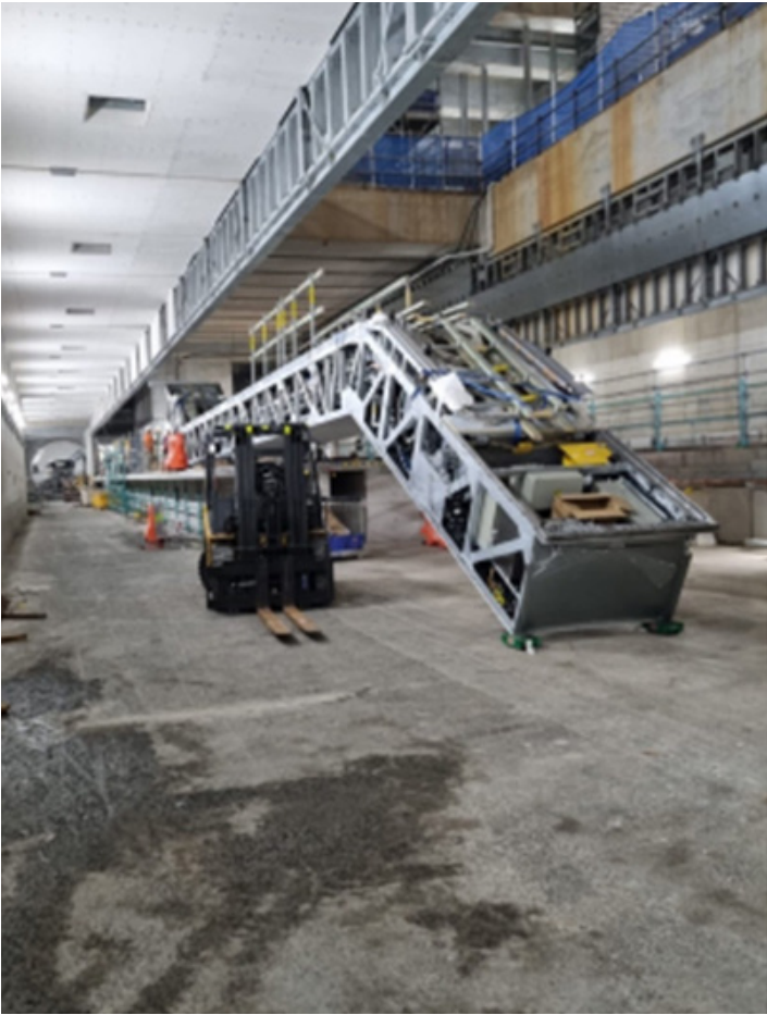
Installation of escalators to the station platform
