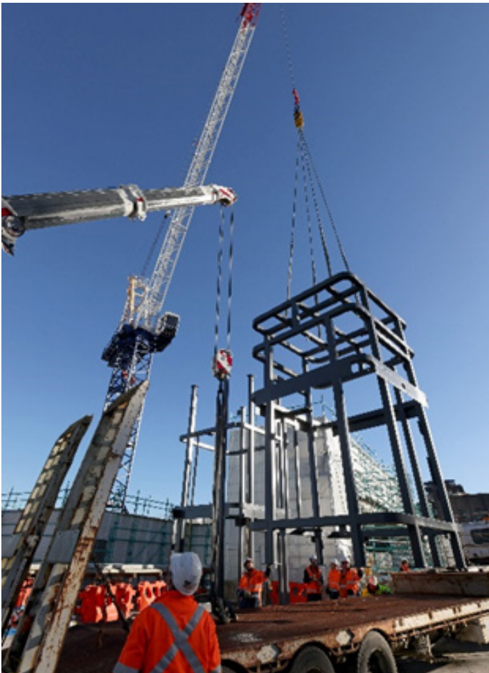
Crane moving structural steel for the lifts
