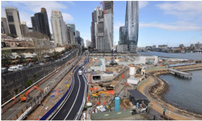
The two alignments of Hickson Road, side by side. Demolition commenced on the Hickson Road alignment in July (far left), while traffic has been diverted to the temporary alignment.
