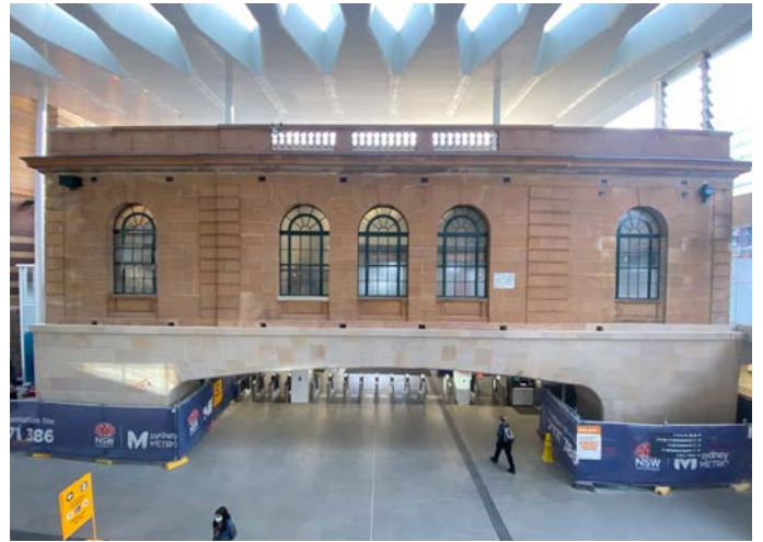
The archway under the Central Electric Building
