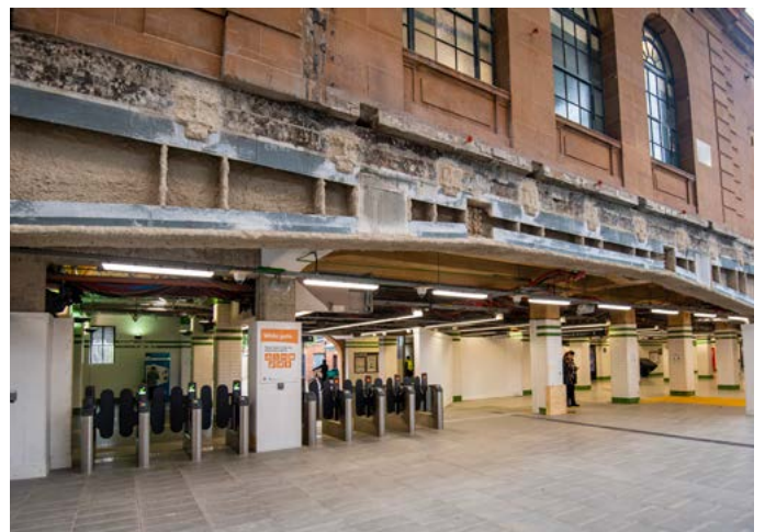
The archway showing the concrete beam before sandstone cladding is installed
