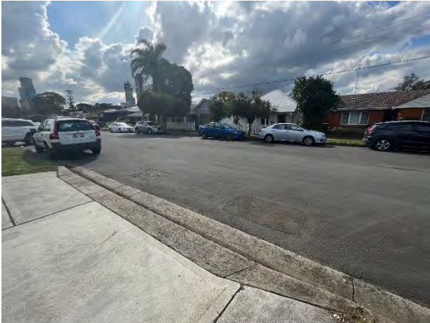
Photo 5.3 General location of proposed boreholes GALC-BH32, GALC-BH33 and MW20. View north across Oak Street. Image Source: Umwelt 2022
