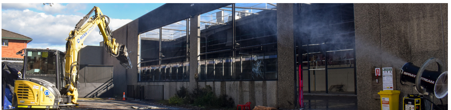
Sprinkler systems were used extensively during demolition work at St Marys to suppress dust.
