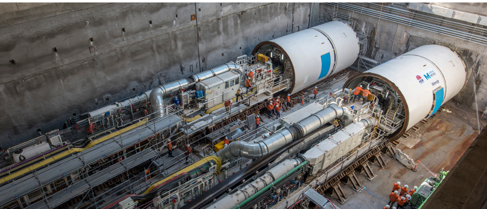
Four tunnel boring machines will build the Sydney Metro - Western Sydney Airport tunnels.
