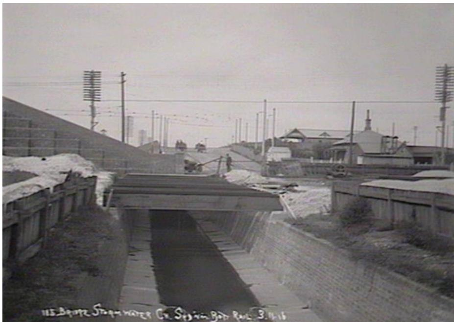
Figure 16. Bridge, stormwater channel, Sydenham–Botany rail, 3 November 1916. View shows the 1898 stormwater channel, the Marrickville Road railway embankment wall (left), the Sydenham station concourse buildings (top right) and the buildings that occupied the area adjacent to the Bankstown line between Gleeson Avenue and Marrickville Road (SLNSW image 221599).
