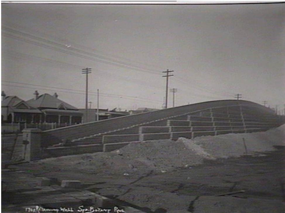
Figure 10. Construction of retaining wall adjacent to Railway parade, Sydenham n.d. (1916)
