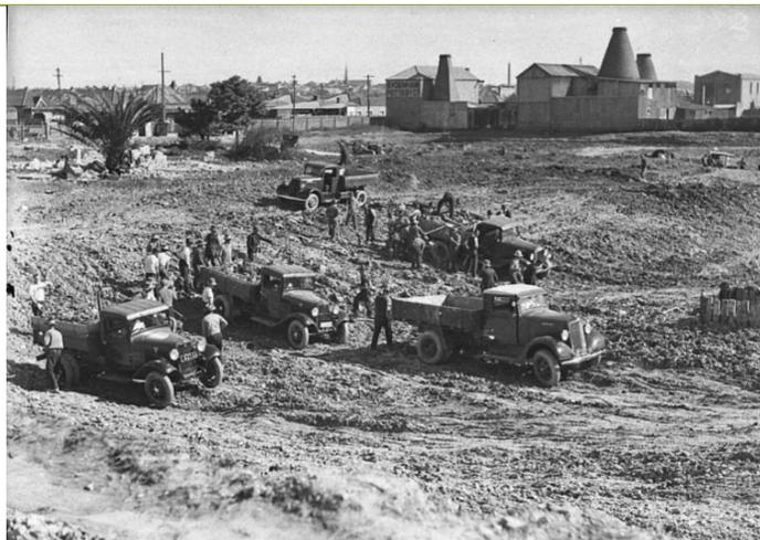
Figure 24. Works at Sydenham 1935. Excavation of the Sydenham Drainage Pit looking northwest towards the Garden Street/Shirlow Street intersection. The Sydenham Pottery Company at top right (SLNSW 81937).
