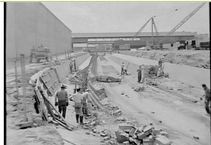
Figure 25. Storm drain, Sydenham 1965. The image shows the removal and replacement of the c.1898 brick channel by the extant concrete channel adjacent to Sydney Steel Company, looking north (SLNSW Government Printing Office 2—26989).
