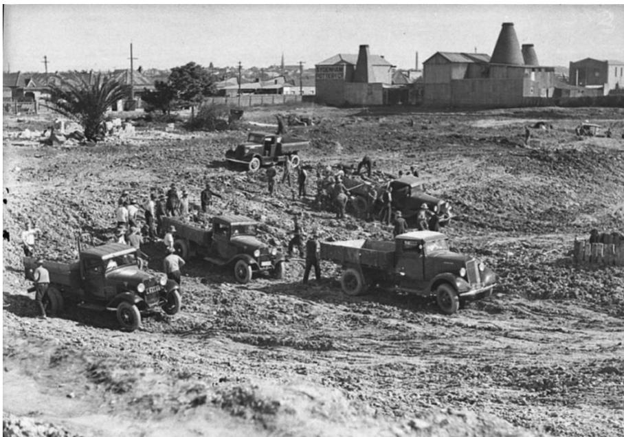
Figure 18. Works at Sydenham 1935. Excavation of the Sydenham Drainage Pit looking northwest towards the Garden Street/Shirlow Street intersection. The Sydenham Pottery Company at top right (SLNSW 81937).
