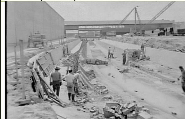
Figure 41. Storm drain, Sydenham 1965. The image shows the removal and replacement of the c.1898 brick channel by the extant concrete channel adjacent to Sydney Steel Company, looking north (SLNSW Government Printing Office 2—26989)
