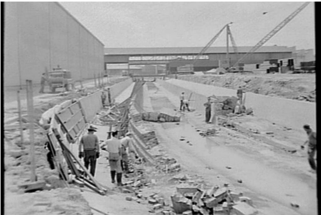
Figure 20. Storm drain, Sydenham 1965. The image shows the removal and replacement of the c.1898 brick channel by the extant concrete channel adjacent to Sydney Steel Company, looking north (SLNSW Government Printing Office 2—26989).
