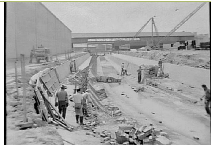
Figure 25. Storm drain, Sydenham 1965. The image shows the removal and replacement of the c.1898 brick channel by the extant concrete channel adjacent to Sydney Steel Company, looking north (SLNSW Government Printing Office 2—26989).
