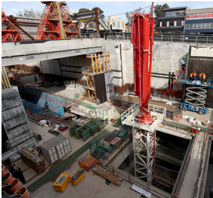
Building of the perimeter wall (waterproofing covered by steel reinforcement prior to concrete being poured to create the wall)
