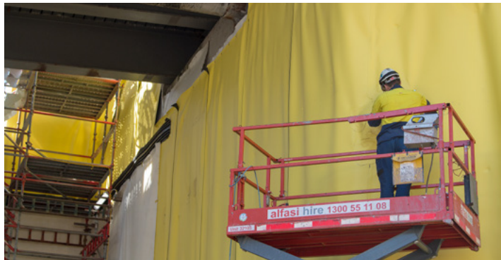
Bright yellow layer of water proofing that sits behind the perimeter
