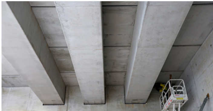
Structural pre-cast beams that make up the concourse level of the station
