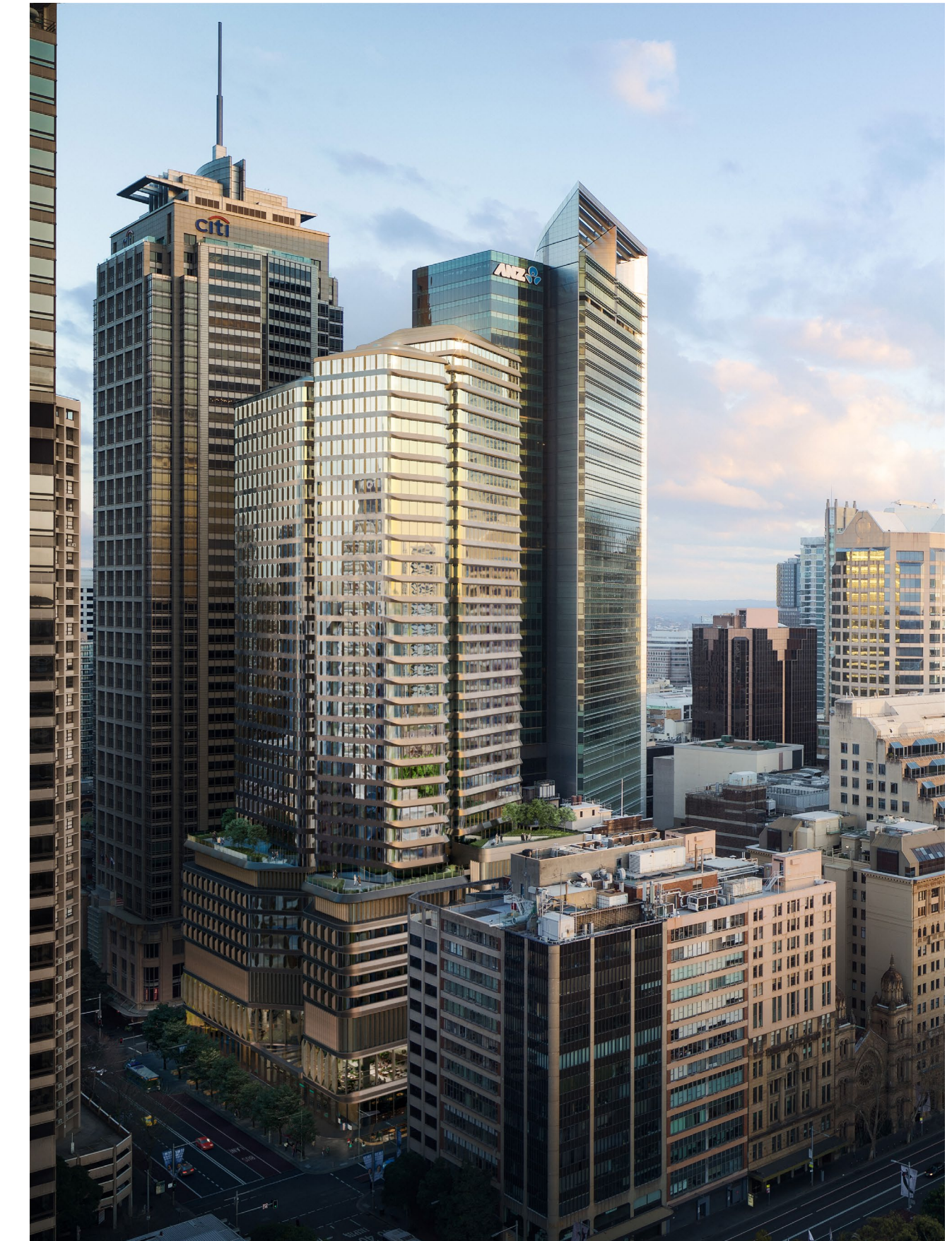
An artist's impression of Pitt Street North over station development looking east
