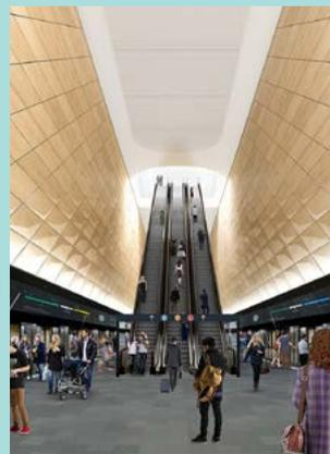
The new walls in the Sydney Metro platform area makes reference to the heritage masonry fabric. The cladding adopts a diamond-shaped geometry in contrast to the traditional stonework. The wall panelling functions as a wayfinding element where the sandstone-coloured panels literally point upwards in the direction of the journey towards the upper level concourses and conceptually towards the clock tower.
