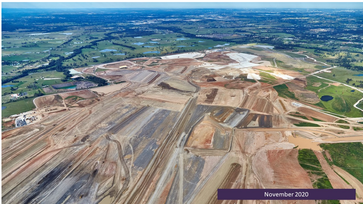
Figure 5-1 Major Earthworks progress on WSA CIZ
