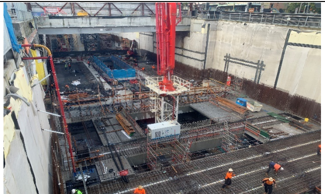
Level B2 view South – Slab Steelfixing and formwork
