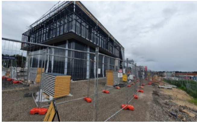
SMTF – S Maintenance Building - structural steel, roof mesh installation and cable containment works ongoing.
