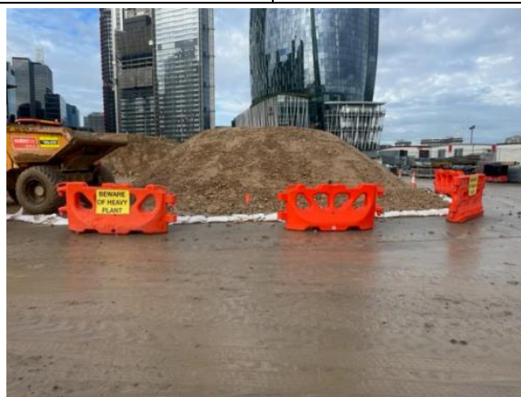
Controls were in place around the base of the Rozelle interchange tunnelling spoil stockpile.
