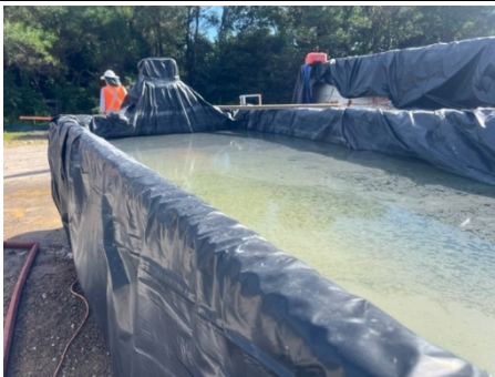
Belmore Triangle, Redman Parade: Vacuum truck slurry storage (to be disposed offsite as liquid waste), and dewatering of Pits 5 & 9 to land under a water monitoring program
