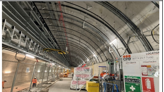
Eastern cavern: Structure for upper cladding panels
