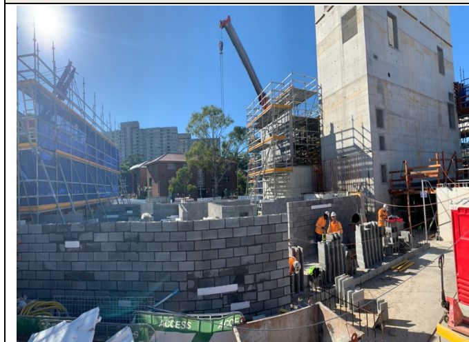
Ongoing FRP and recent commencement of blockworks (including block cutting) on Ground Level
