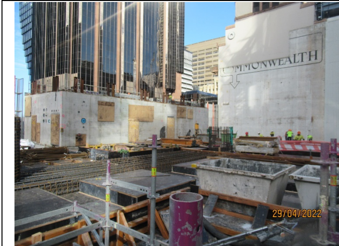
Martin Place North – FRP for concrete slab and beams.
