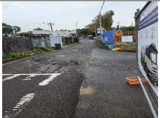
Dulwich Hill MSB minor sediment and potholes requiring maintenance 27.04.22
