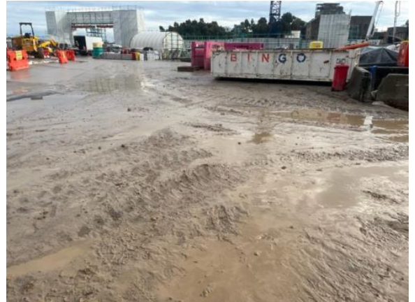
A layer of mud had built up across the hardstand, increasing the risk of sediment-laden runoff and tracking offsite
