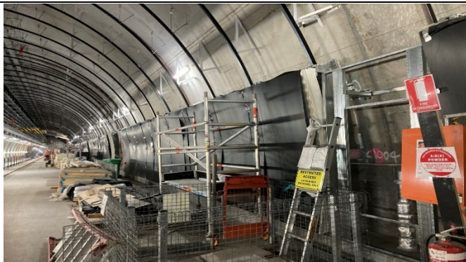
Western Platform, lower GRC cladding
