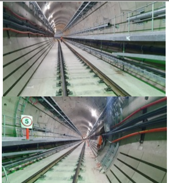
Northern Hub - Tunnel (Up) - Sound proofing, services (temporary/permanent), HV cabling, walkway installation and extent of track installed upto Victoria Cross Station.
