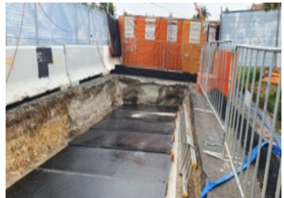
Canterbury to Campsie BPS - Joint Bay worksite (Anzac St)
