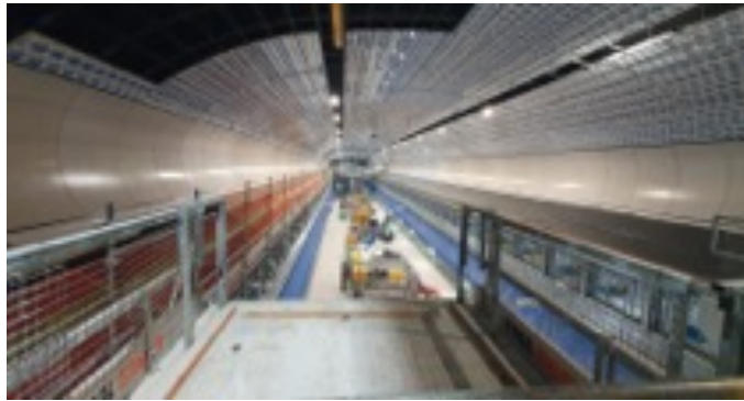
Cavern: Installation of cladding and GRC panels progressing on Cavern roof.
