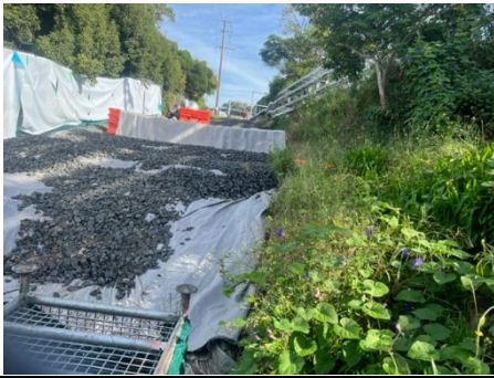
Ewart Street, Dulwich Hill: Establishment and improvement of ERSED controls
