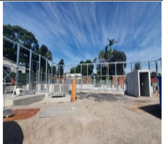
Dulwich Hill TSS - Steel installed for future façade panels.
