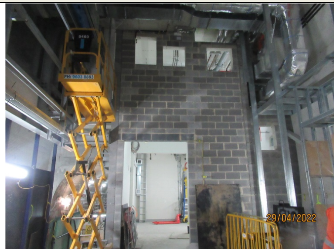
Platform Caverns – Fit out and block wall construction for back of house operations
