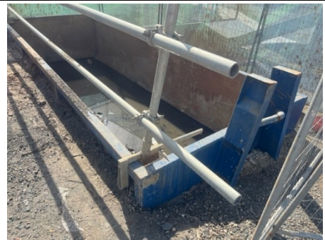
Belmore Triangle, Redman Parade: Vacuum truck slurry storage (to be disposed offsite as liquid waste), and dewatering of Pits 5 & 9 to land under a water monitoring program
