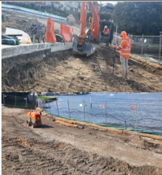
Blues Point Access Site - Trimming and compaction works underway (lower end of site, near Harbour side).
