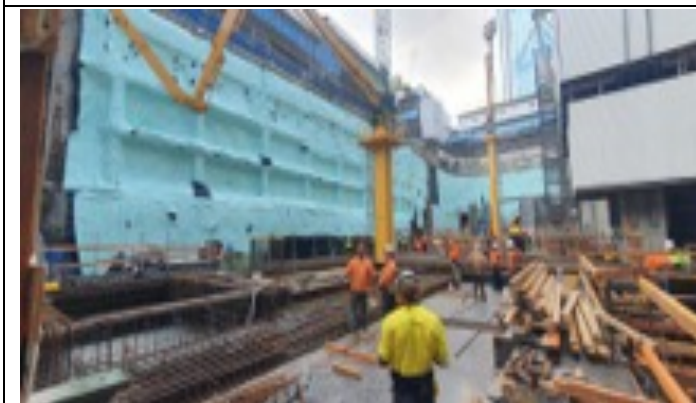
Victoria Cross South: Waterproofing works progressing along on the Western side of Station and adits.
