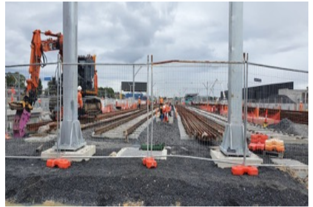
SMTF S – Rail and sleeper install ongoing.
