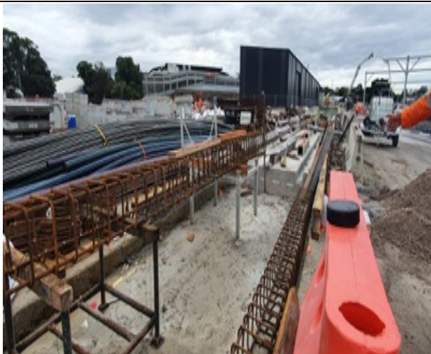
SMTF – S - Track slab FRP works ongoing.
