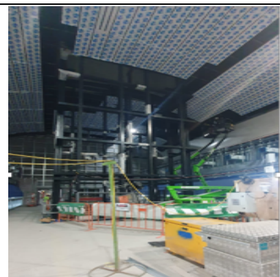
Cavern: Lift framework installation progressing
