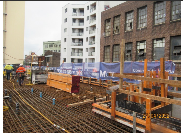
Preparation for concrete pour on roof of the Eastern Entrance
