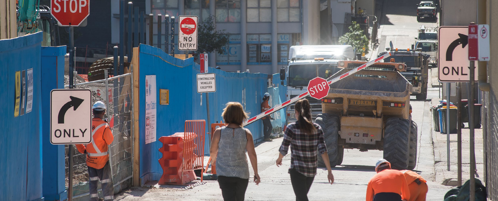
Crows Nest Station at Hume Street.
