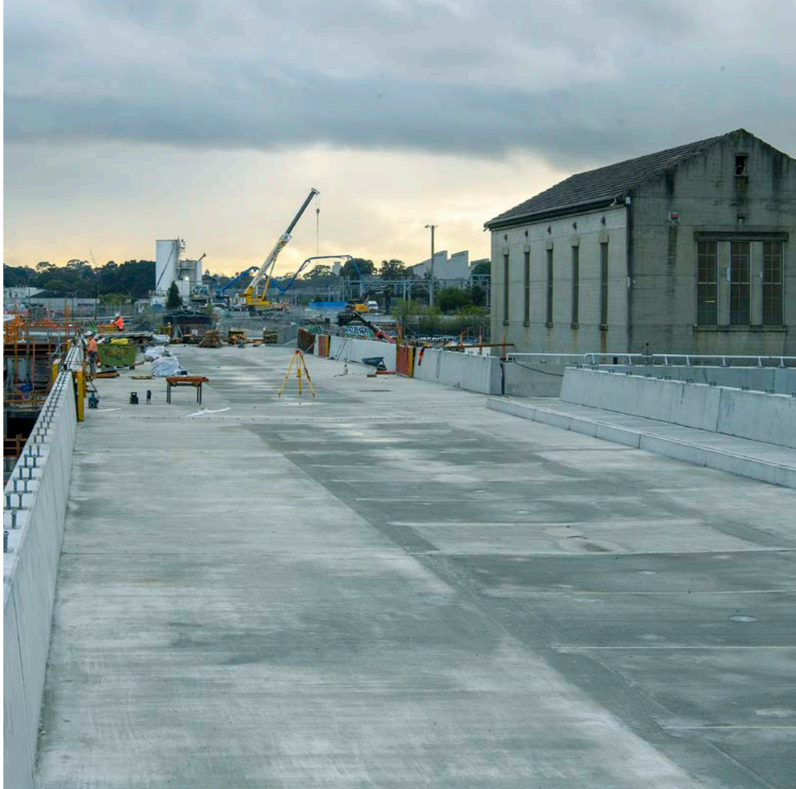
Construction of the new aqueduct over the existing heritage-listed Sydenham Pit while retaining the existing heritage listed pump station.
