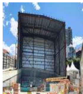
Blues Point Access Site - Preparatory works and scaffolding in progress for demobilisation of site acoustic shed.
