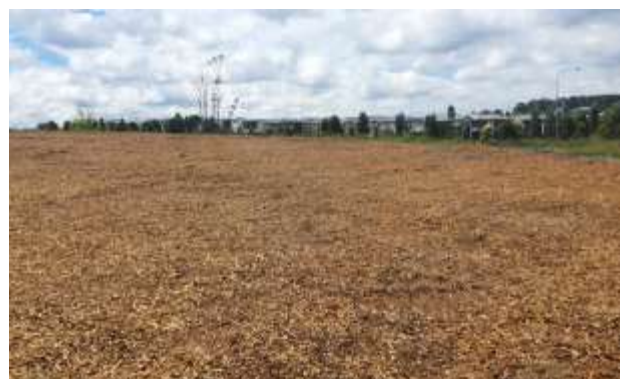
SMTF North – Snake Mountain Ara -Stabilising works are nearing completion with some mulch remaining to be applied and additional ballast to be laid in areas of concentrated flow
