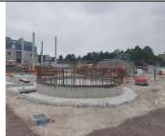
SMTF S - Water Treat Plant (WTP) for operational phase progressing. Preparatory works for concrete pour for Emergency Water Tank.
