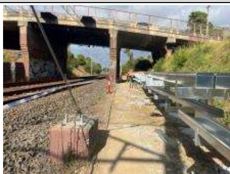
Moreton Street, Punchbowl: Cess drainage pits were unprotected in the vicinity of the GST installation work area
