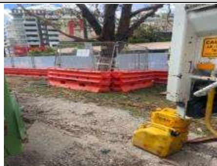
Bankstown MSB Site: Two jerry cans of diesel were stored without secondary containment
