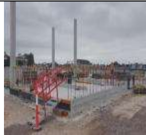
SMTF S - Water Treat Plant (WTP) for operational phase progressing. Preparatory works for concrete pour for Emergency Water Tank.
