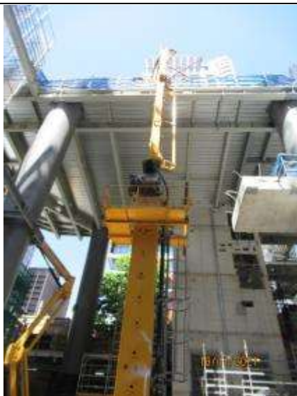
10 Martin Place North – Concrete pump placing concrete in hollow steel columns
