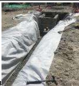
SMTF S - Stabling Yard – excavation for inter tack drainage underway. Drain (second photo) within future stabling yard footprint was protected.
