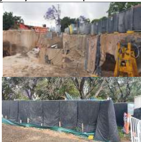
Canterbury TSS - Noise blankets remain installed on Hutton St side. No high-noise works being undertaken at the time of the inspection.
