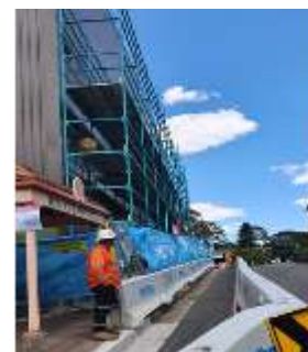
Blues Point Access Site - Preparatory works and scaffolding in progress for demobilisation of site acoustic shed.
