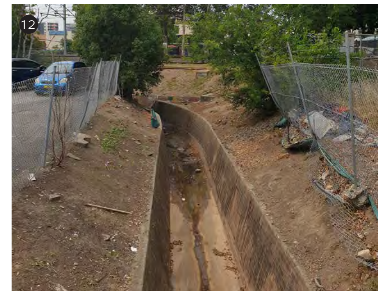
Sydney Water culvert
