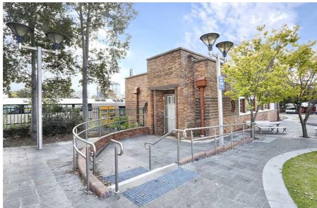
Figure 4.12 Parcels Office present day condition - as viewed from South Terrace
