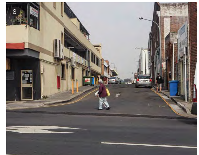
Lack of pedestrian crossing at Stewart Lane
