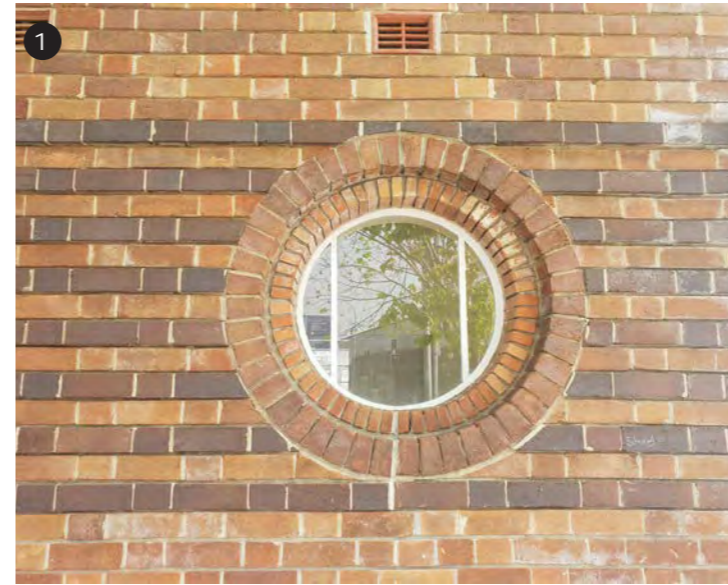
Detail of Heritage Parcels Office
