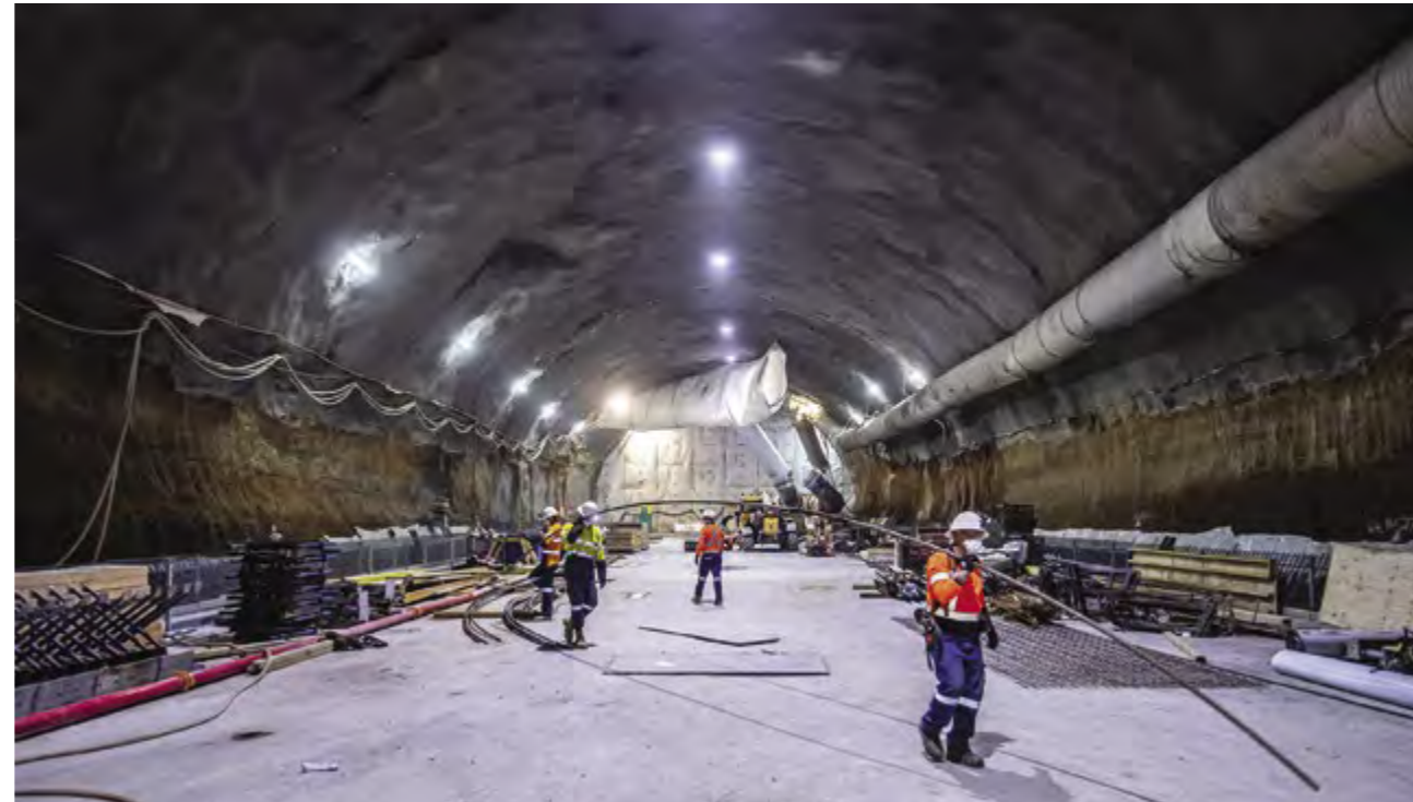
Sydney Metro's crossover cavern at Barangaroo.
