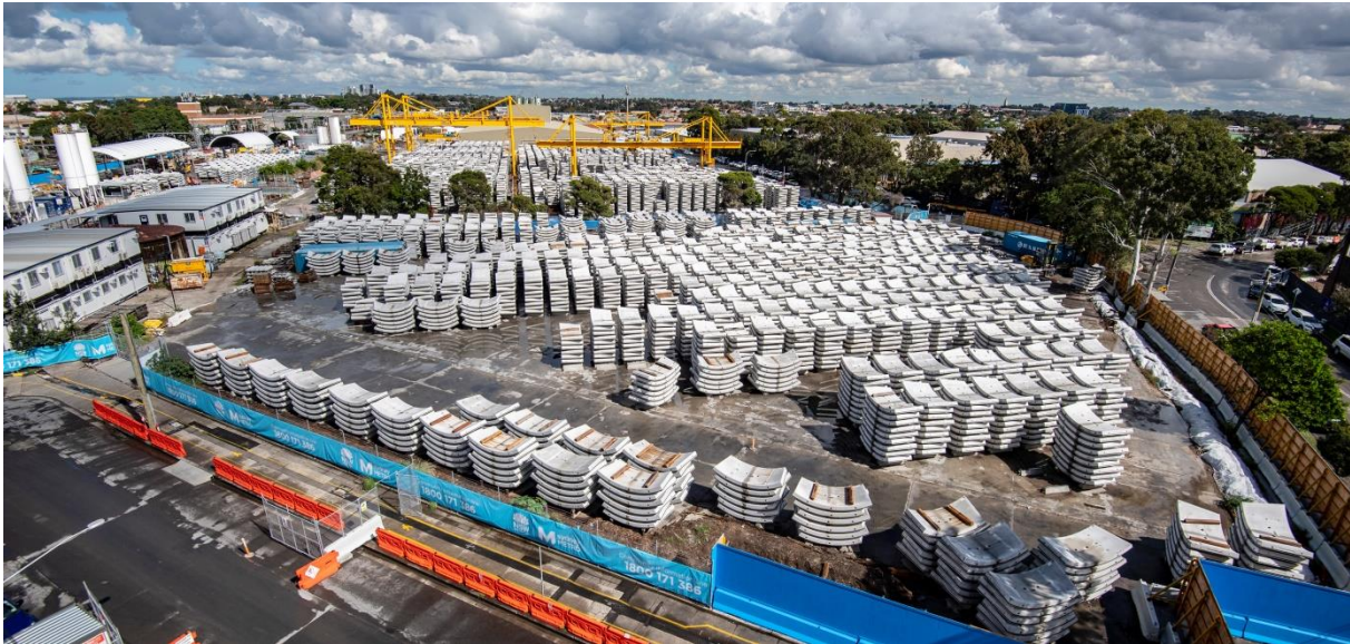
Figure 4-24 Photo of the tunnel segment storage area at Marrickville for the Sydney Metro City & Southwest project (indicative example of the proposed facility within Western Sydney International)
