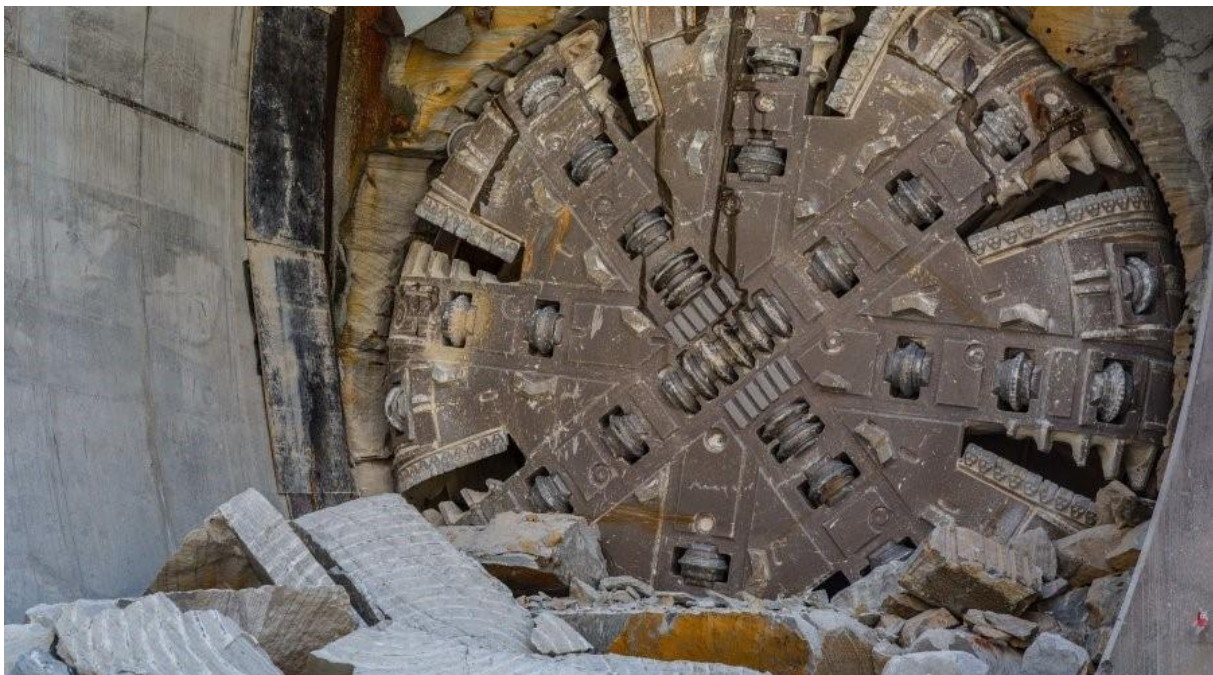
Figure 4-23 Photo of a tunnel boring machine at Epping Station on the Metro North West Line
