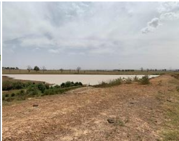
Photo 5.26 Constructed agricultural dam
