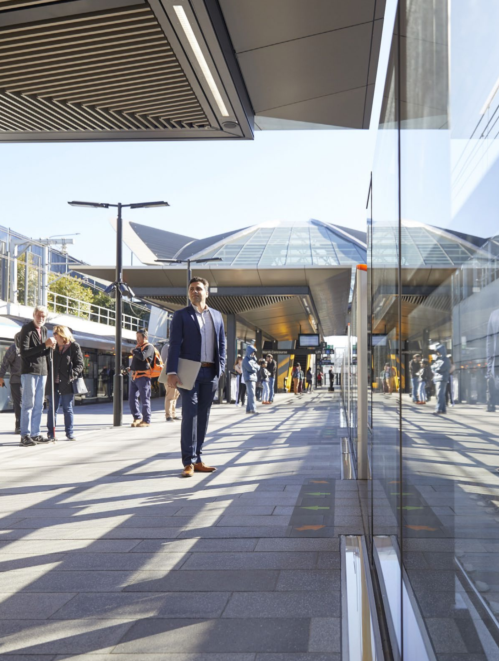
Bella Vista Station, Metro North West Line.
