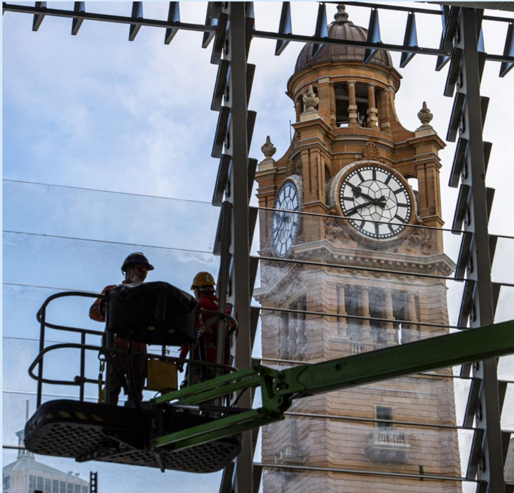
Northern Concourse at Central Station.
