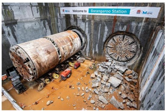
Tunnel boring machine Mum Shirl (right) breaks through at the Sydney Metro Barangaroo station site joining tunnel boring machine Nancy inside the station box, January 16, 2020.
