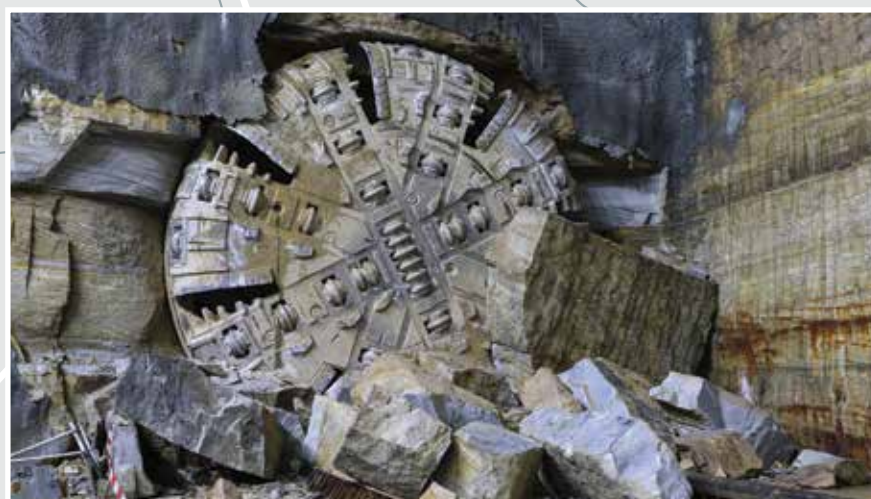
TBM2 Florence break-through at Showground, June 2015
