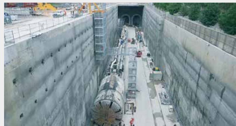
Following the first break-through, TBM1 Elizabeth traverses the Norwest Station site, February 2015
