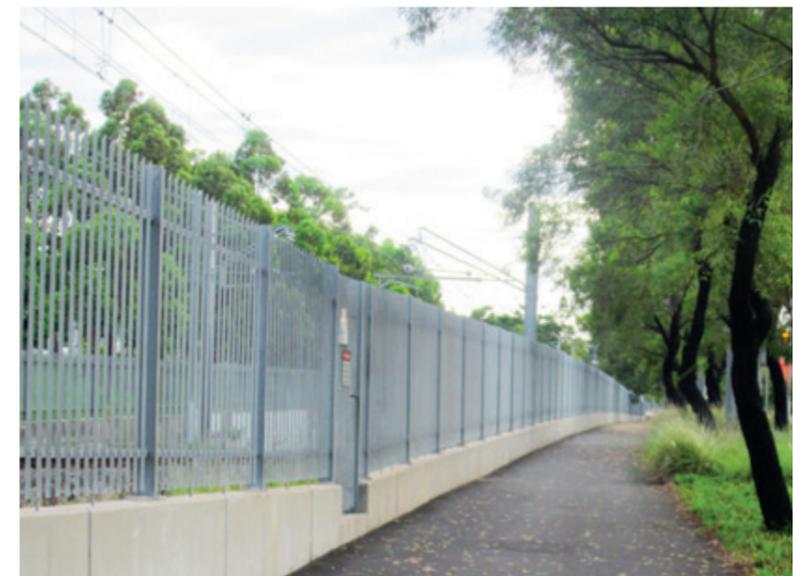
Homebush, Sydney. Rail corridor security fences should be robust, easily maintained, modular systems that are readily integrated with other urban design elements such as retaining walls.
