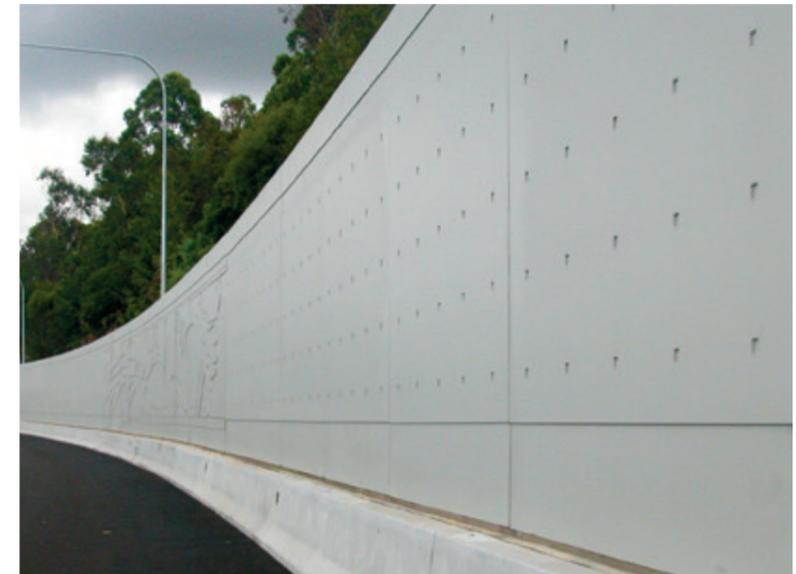
Gore Hill Freeway, Sydney. Provide retaining walls that are topped out by a consistent concrete capping beam.
