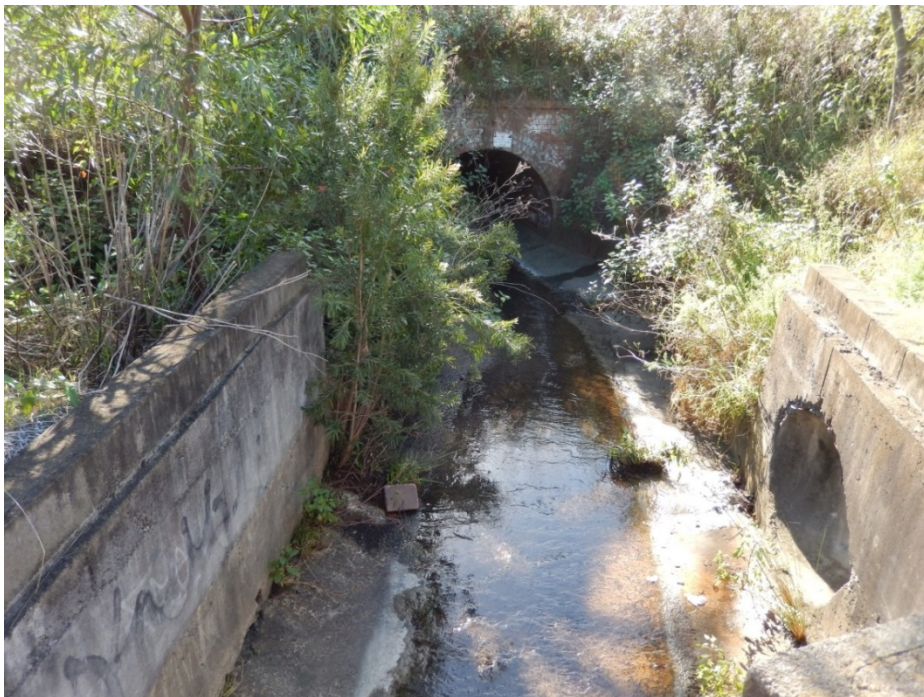
Figure A.8 Culvert under rail corridor near Belmore Sportsground
