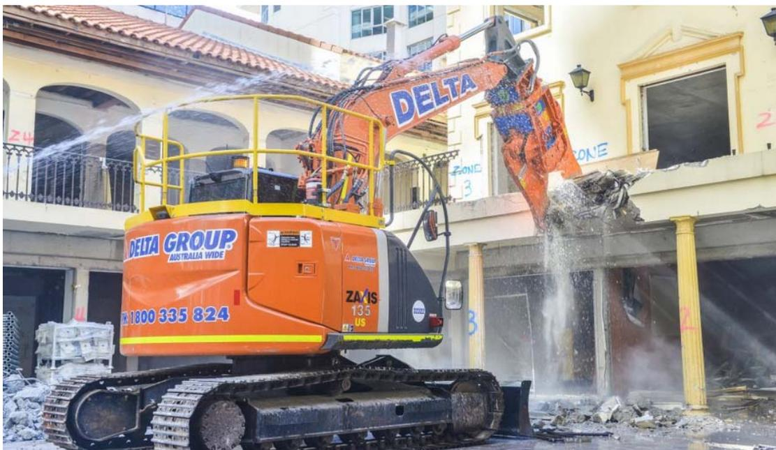
Figure 5: A Pulveriser being used for Demolition at the Victoria Cross Station Site
