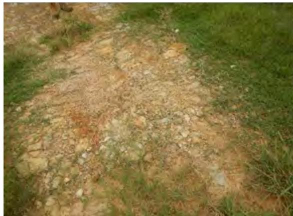
**Figure 39: Sandstone cobbles within backfill layer**
