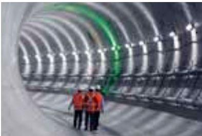
Figure 17: A modern railway tunnel in construction. See more at: https://www.sydneymetro.info/tunnelling
