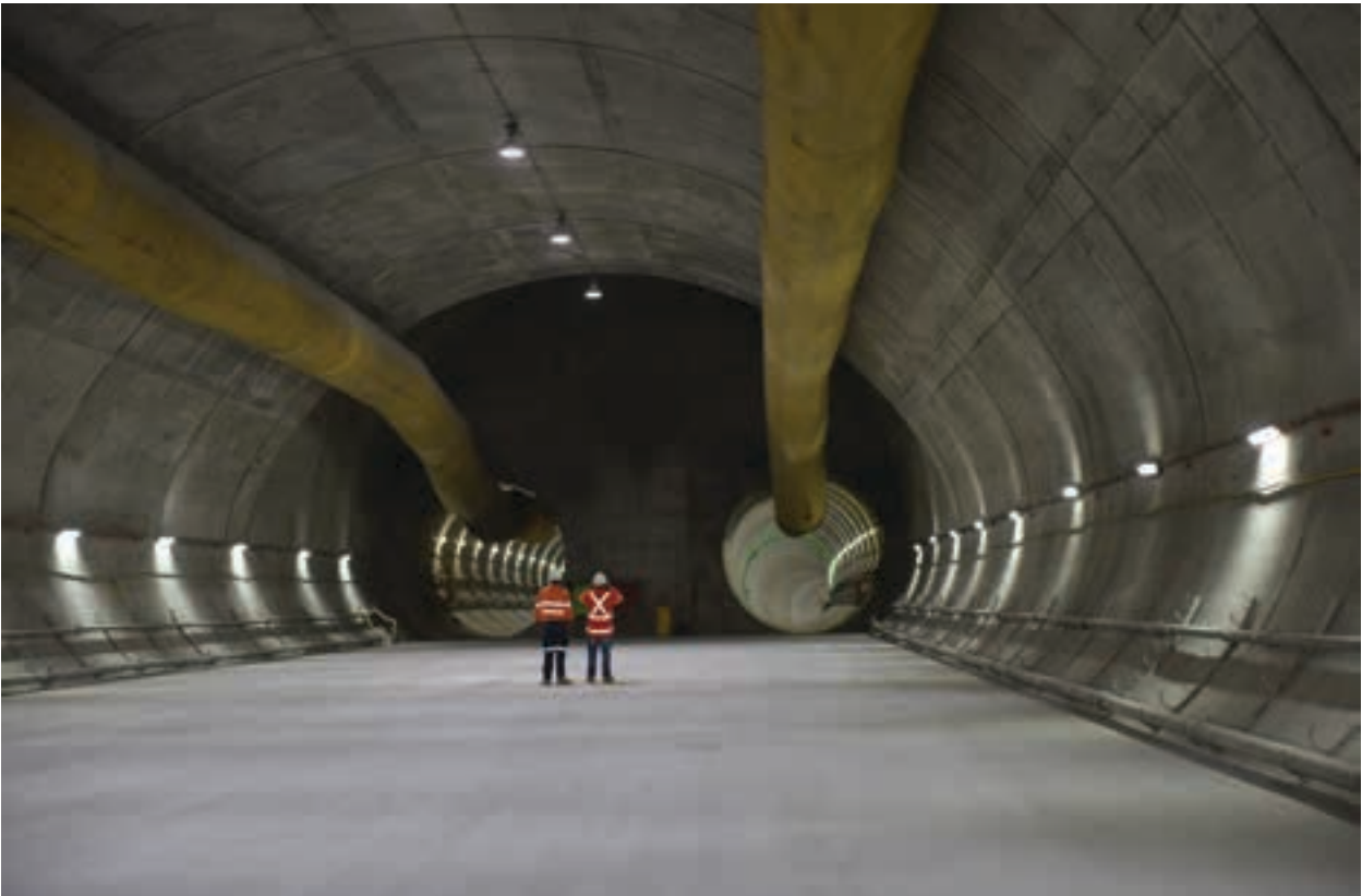
Figure 15: Hills Showground tunnel and Castle Hill crossover tunnel, May 2016.
