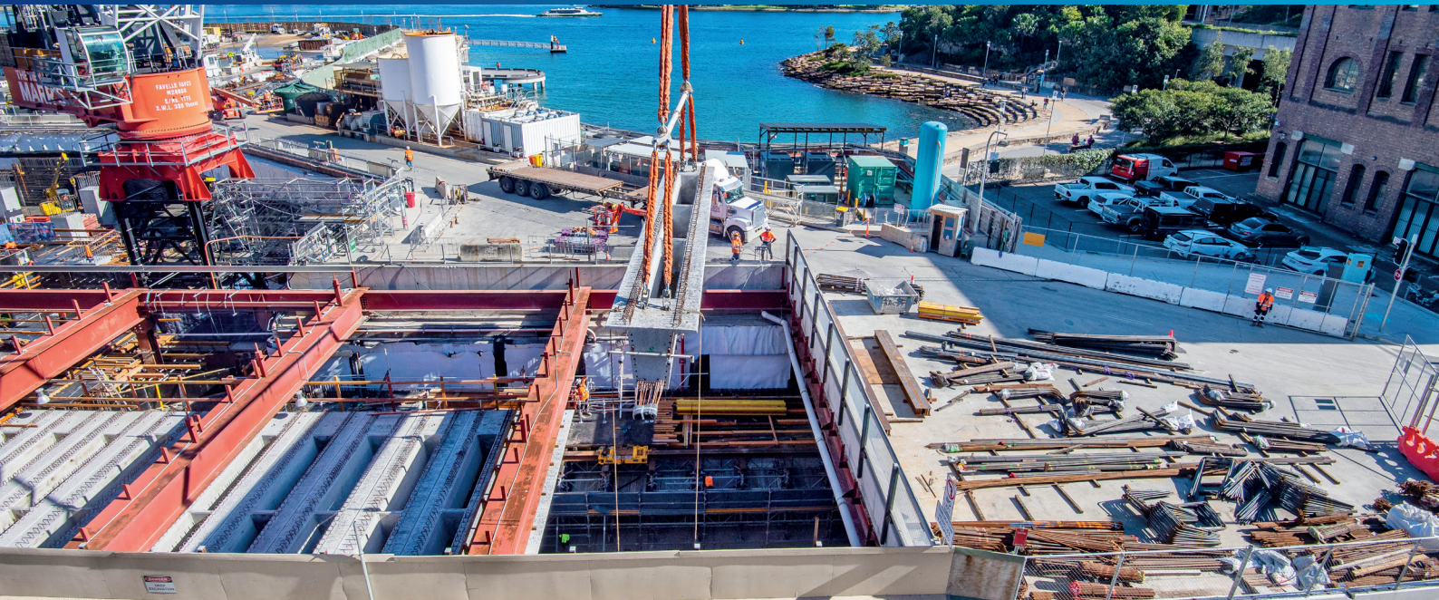
Lifting one of the pre-cast roof beams into place
