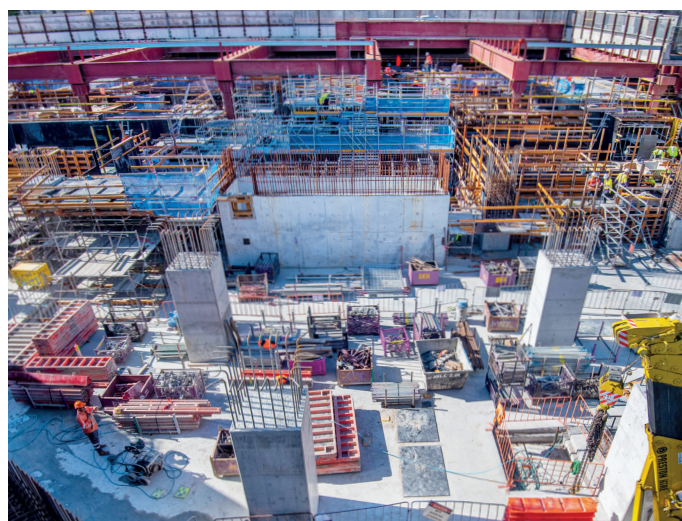
Scaffolding and steel reinforcement dominate at the Barangaroo Station site
