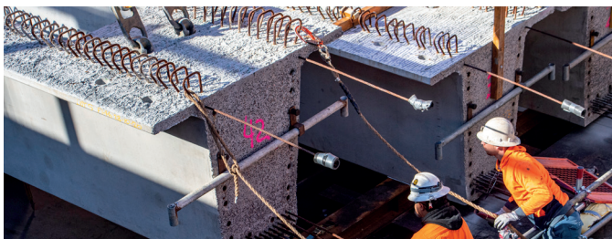
Workers guide a roof beam into place using the customised sliding system
