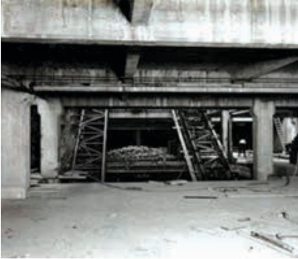
Figure 22: Wynyard Station: erecting the escalators, 1932.
