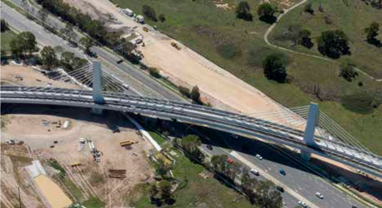
Figure 24: The completed Sydney Metro railway bridge at Rouse Hill, March 2018.
