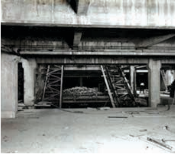
Figure 22: Wynyard Station: erecting the escalators, 1932.
