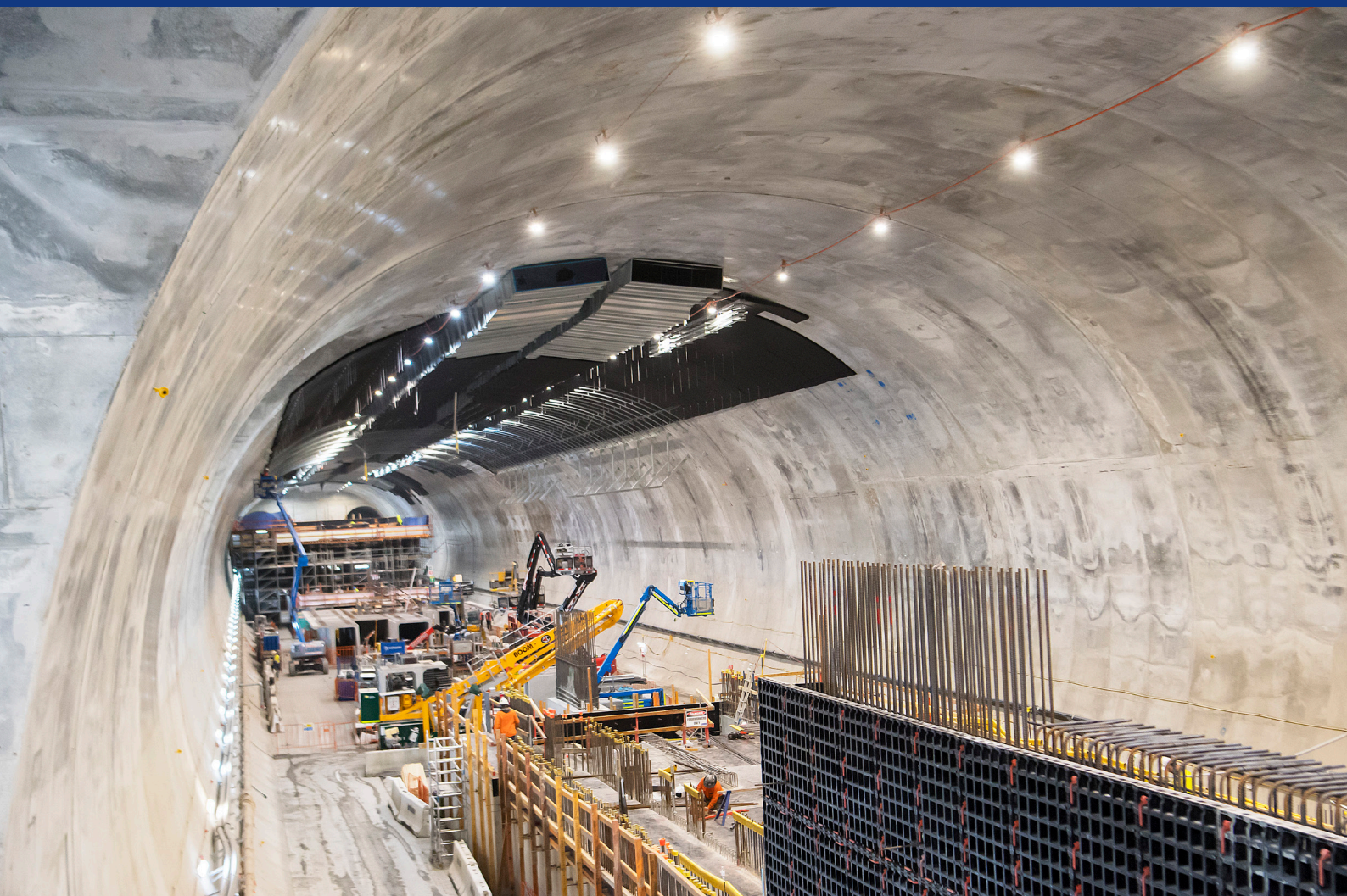
Platform structure taking shape in the Victoria Cross Station cavern.
