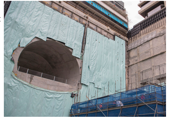
Above: waterproofing in the Victoria Cross South site. Bottom left: station platform structure in the Victoria Cross Station cavern. Bottom right: Victoria Cross North site shaft.
