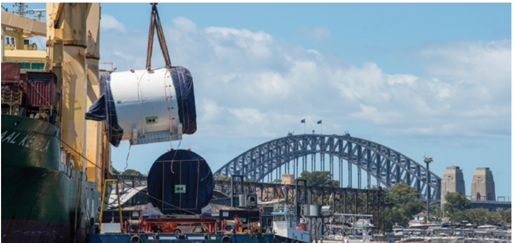
The tunnel boring machine was used to dig twin metro tunnels deep under the harbour, between Barangaroo and Blues Point.
