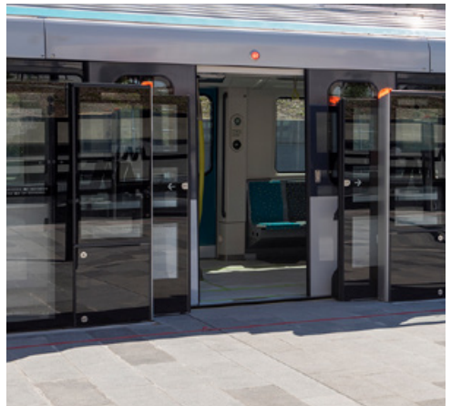
Platform safety screen doors at Tallawong Station.
