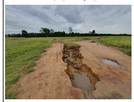
Photograph 16 – Southern Precast Site – Access track washout and dispersive soils (onsite facing east)
