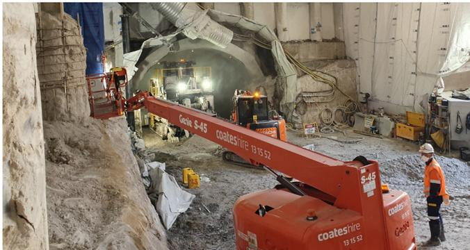
Ventilation dust extraction systems placed at the face of the works.
