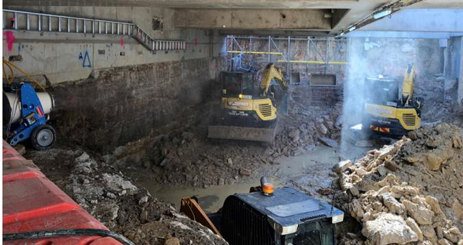
Canon misters used as a method of dust suppression during jack hammering works.
