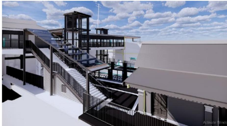
Figure 4.8 New stair, stair canopy and lift in context of heritage roof forms
