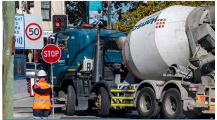
Traffic controller managing concrete deliveries on Hume Street
