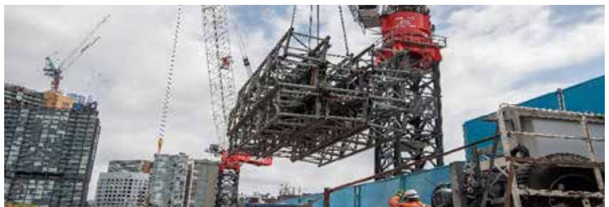
Muscles lifts scaffolding down into the station box
