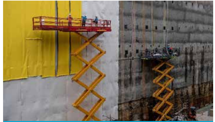
Waterproofing membrane is installed on internal perimeter
