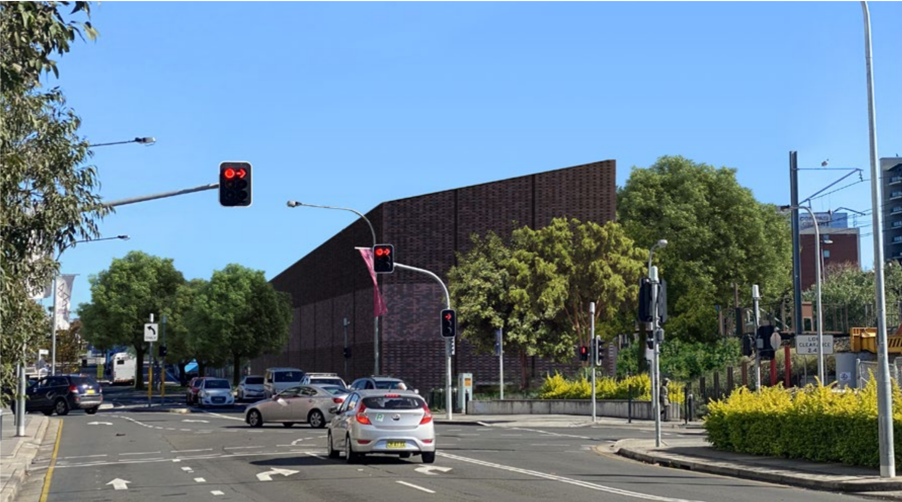
Figure 4.50 View of the Services building from South Terrace
