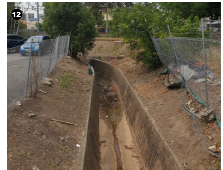
Sydney Water culvert
