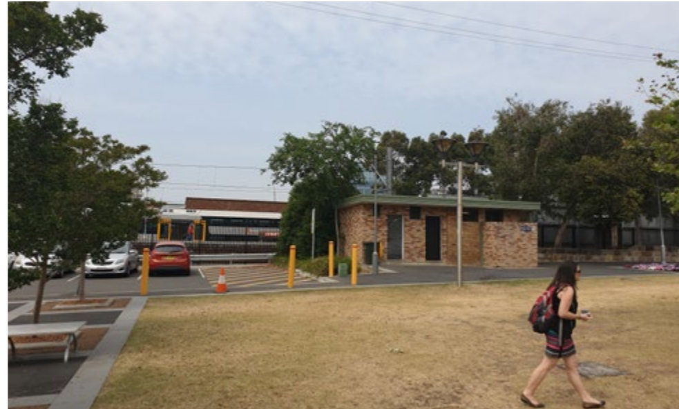
Figure 4.31 Current condition: view from North Terrace
