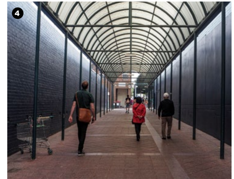
Pedestrian link between South Terrace and Greenfield Parade
