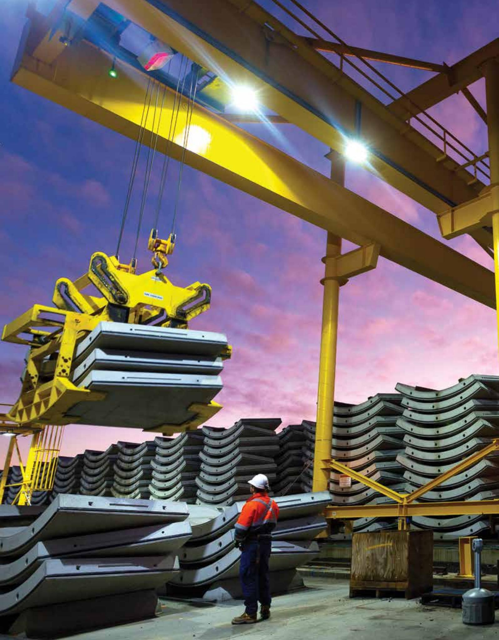
Some of the 100,000 concrete segments used to line the tunnels - June 2015
