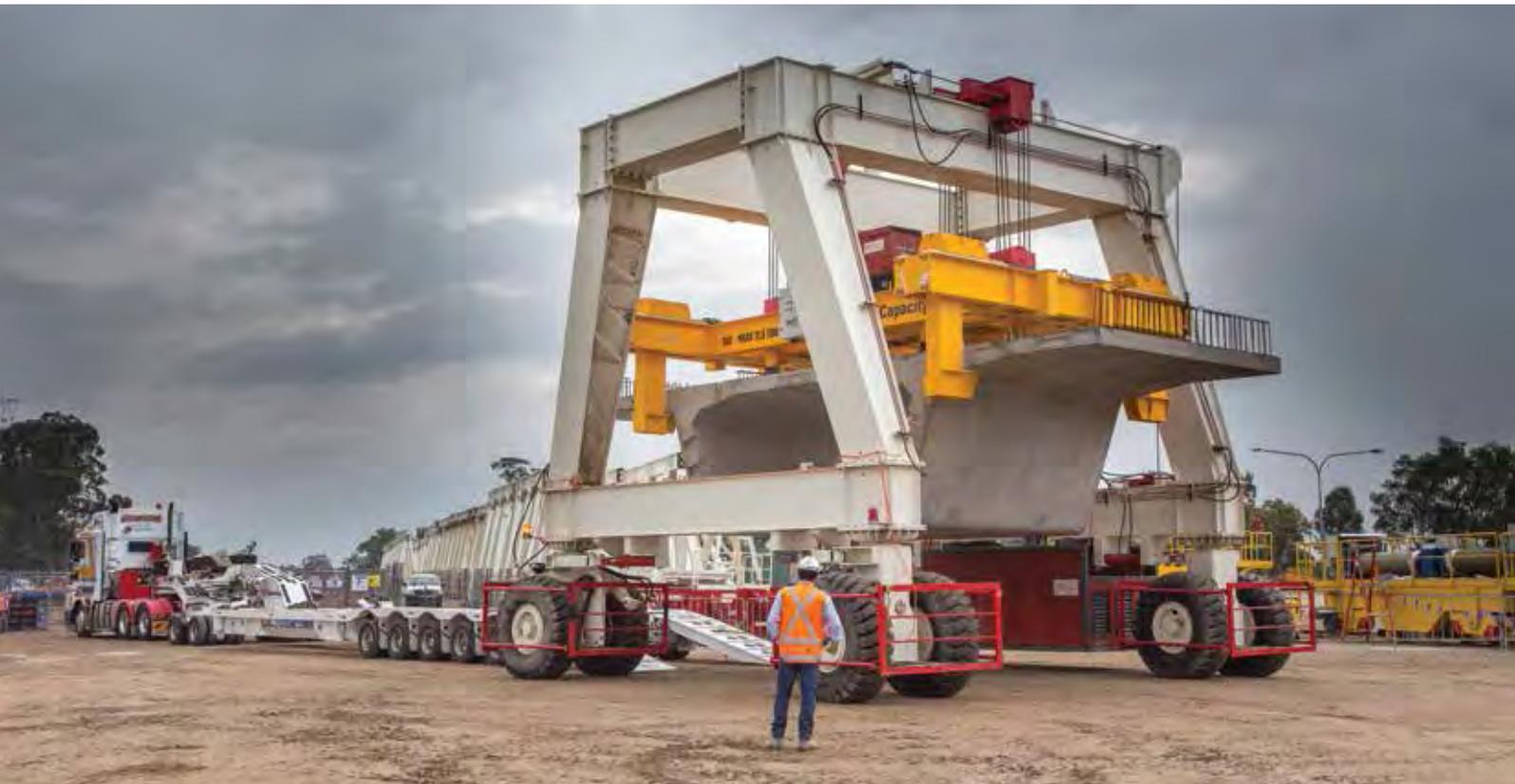
A straddle carrier lifts concrete segments onto a truck for skytrain construction – March 2015
