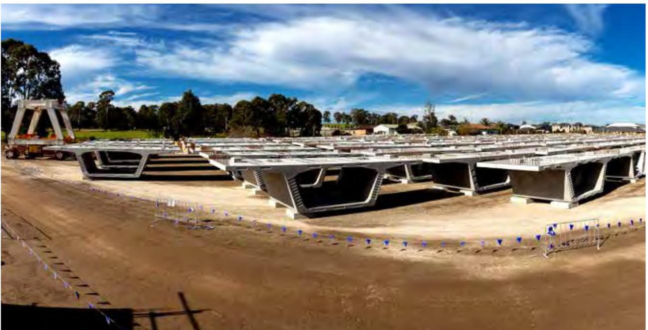
The concrete segments which will form the deck of the skytrain at Rouse Hill - July 2015
