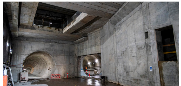
The entrance to the twin Sydney Metro tunnels from the Chatswood dive site
