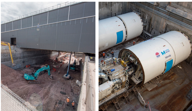
The Chatswood dive where TBMs Wendy and Mabel launched in early 2018
